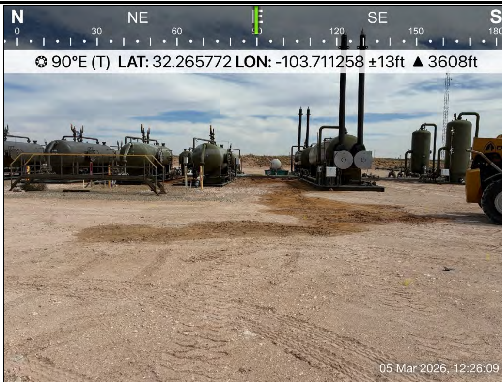
PHOTO 6: Eastern view during site assessment activities for nAPP2606434775. 3/5/2026
