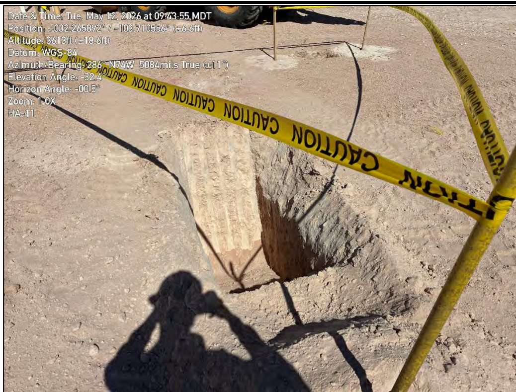
PHOTO 10: Northwestern view during continued delineation activities of nAPP2525125732. 5/12/2026
