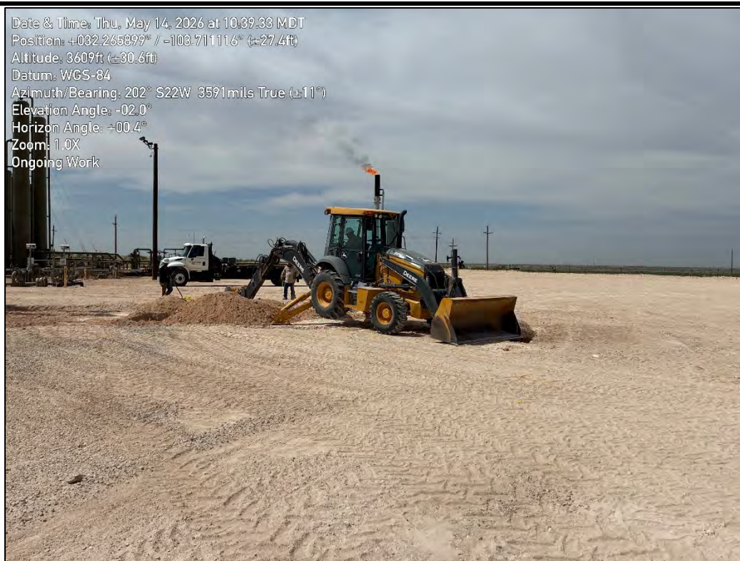
PHOTO 12: Southwestern view during excavation activities. 5/14/2026
