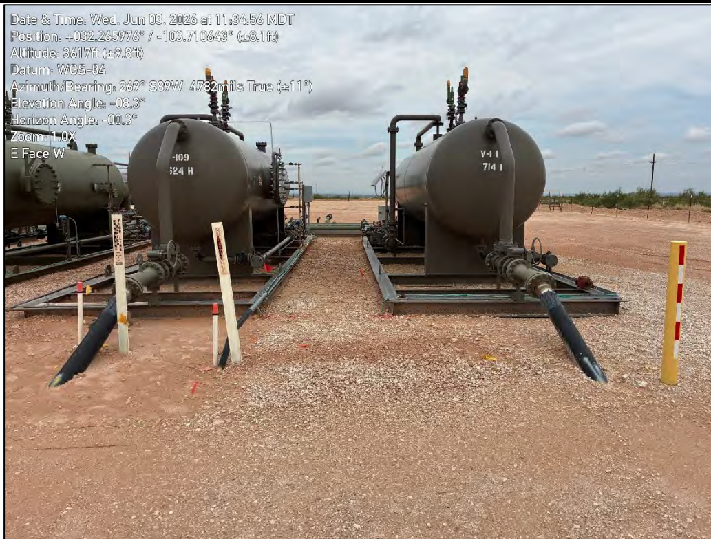
PHOTO 19: Southwestern view following restoration activities. 6/3/2026
