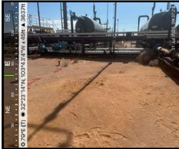
View of area of concern
