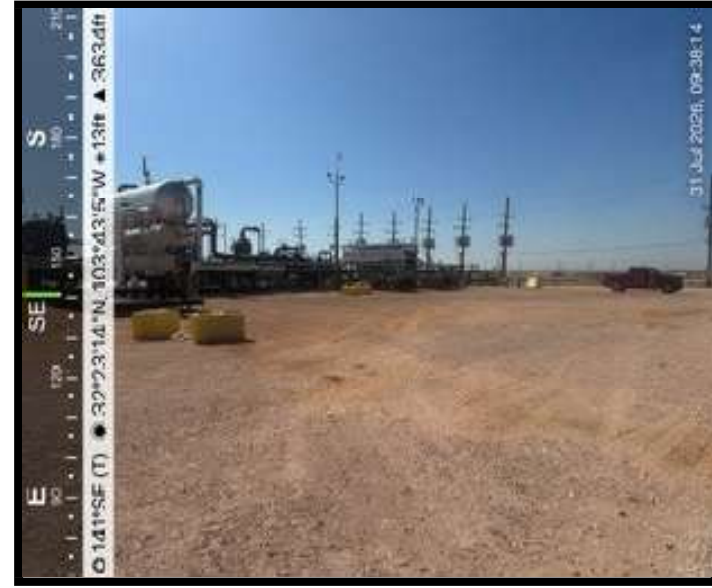
View of area of concern
