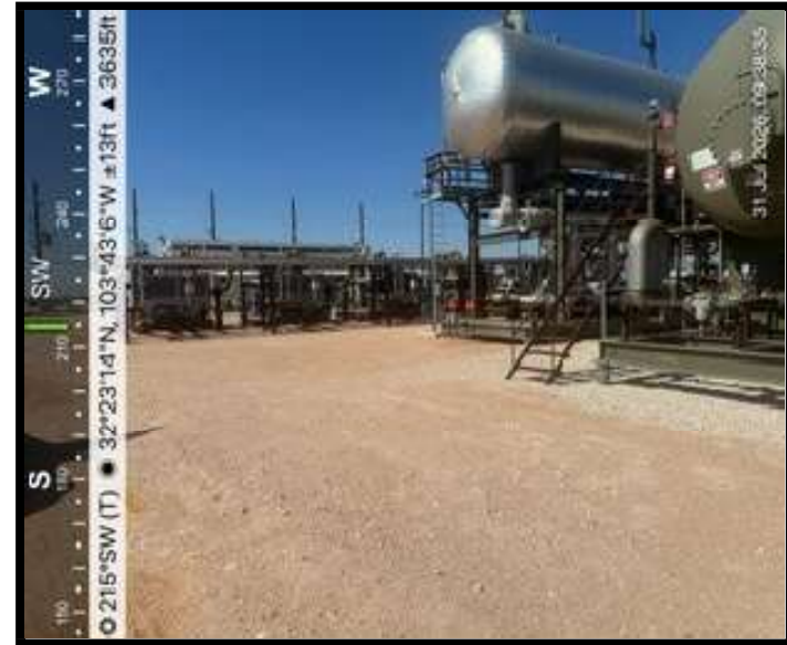
View of area of concern
