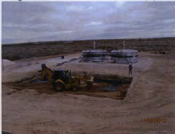
padding the liner with 6 inches of blow sand, facing southwest 11/8/2013
