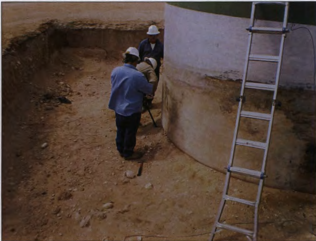
Photograph C– View of soil augering under south tank.
