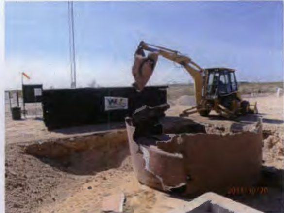
removing the below grade tanks 10/22/2013
