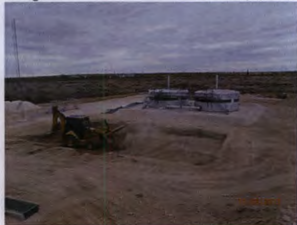
backfilling the excavation with caliche, facing southwest 11/8/2013
