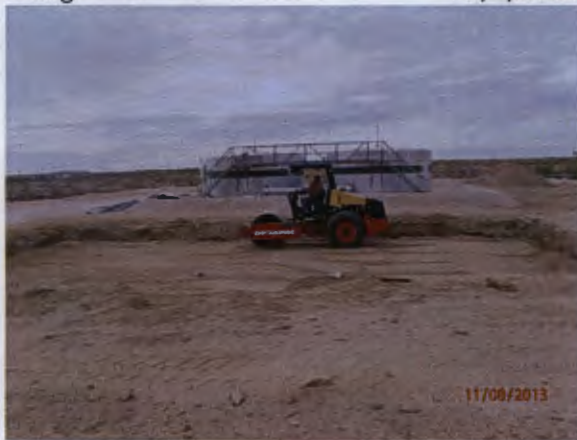
compacting the caliche, facing west 11/8/2013
