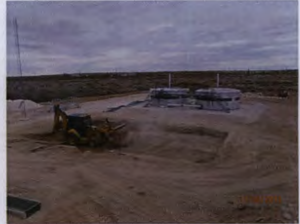
backfilling the excavation with caliche, facing southwest 11/8/2013
