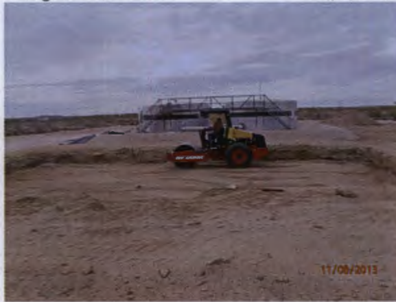
compacting the caliche, facing west 11/8/2013
