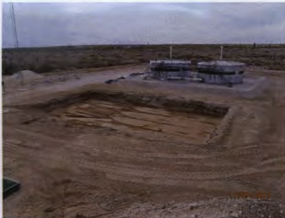
excavation padded with 6 inches of blow sand, facing southwest 11/7/2013
