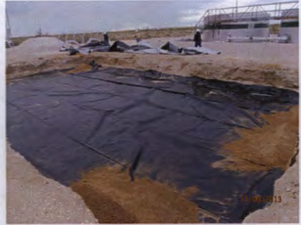
20-mil reinforced liner installed at 4 ft bgs, facing southwest 11/8/2013
