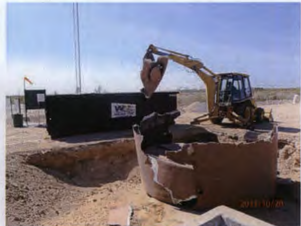
removing the below grade tanks 10/22/2013
