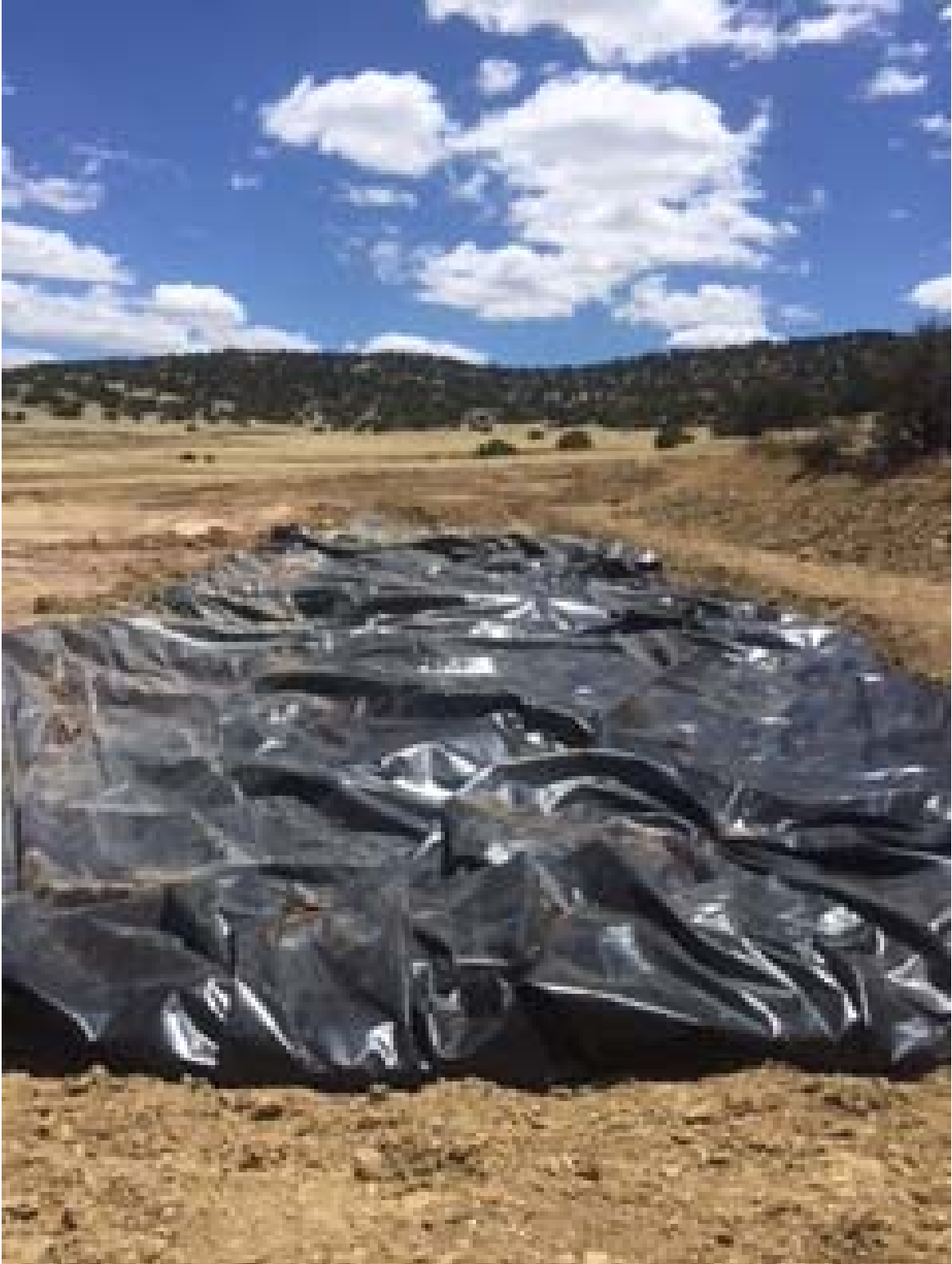
Installation of geomembrane cover over waste material in the lined burial trench.
