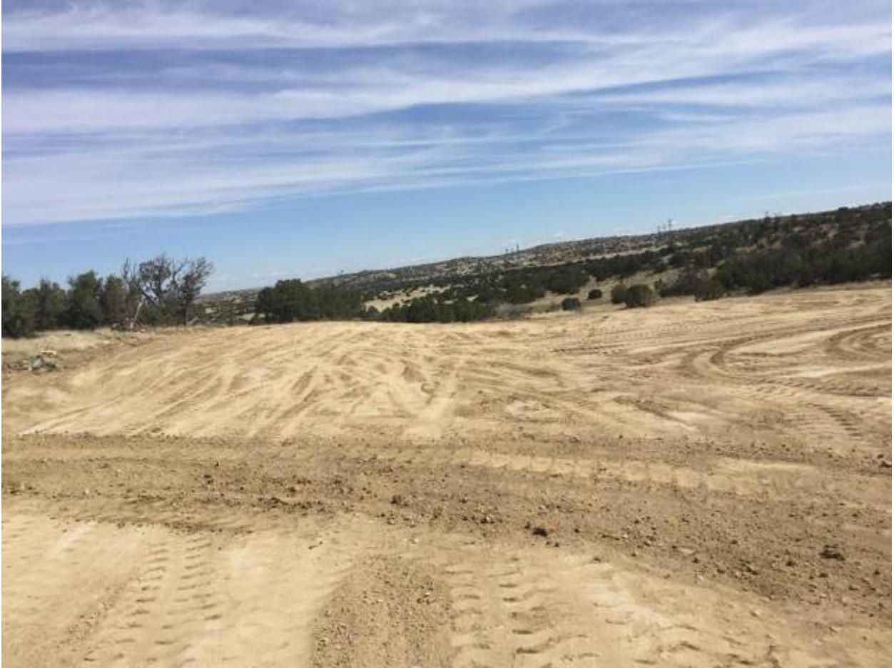
Interim reclamation of CC14 temporary drilling pit area.
