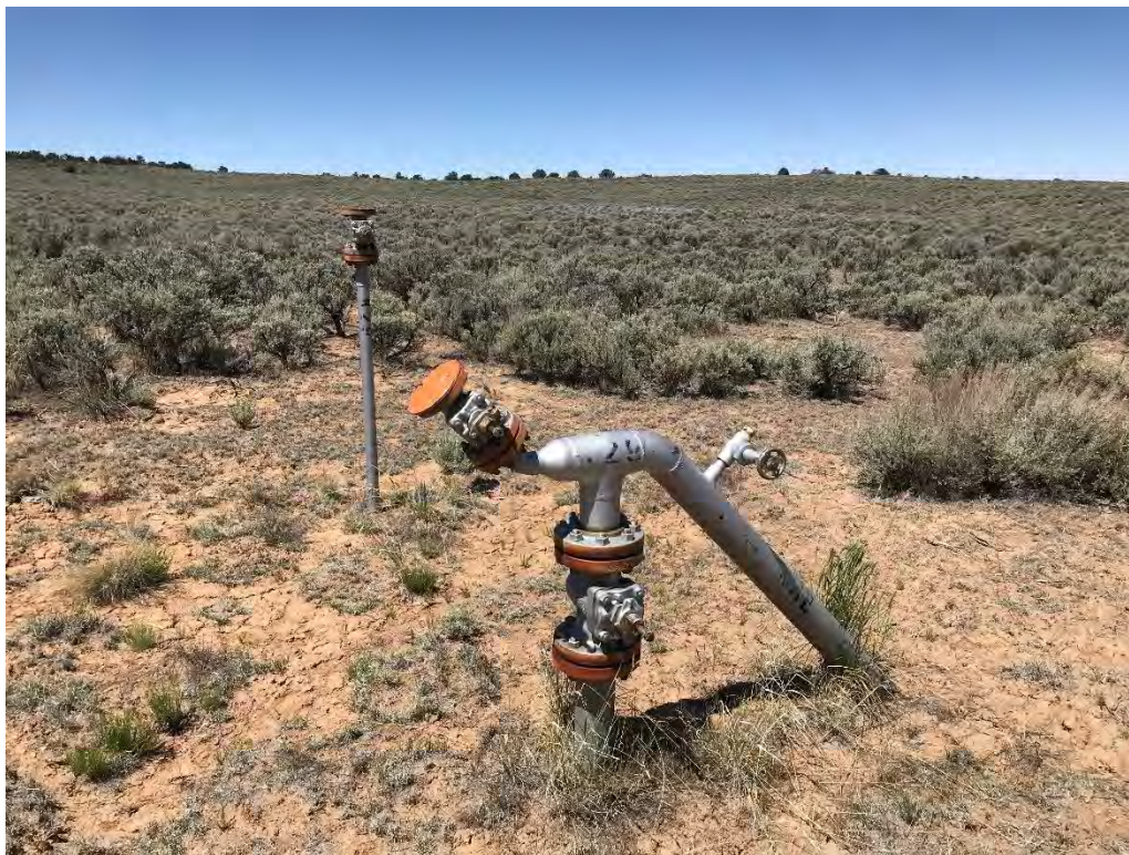
Figure 11. Rincon Unit 068 dogleg and k29 trunk blowdown. BLM requests these appurtenances be removed and pipeline abandoned below grade.
