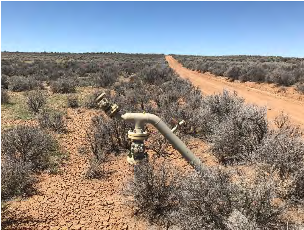
Figure 10. Dogleg at Rincon Unit 202M well-connect pipeline tie-in. Cut and cap below grade as near possible to dogleg on the K29 trunk line.
