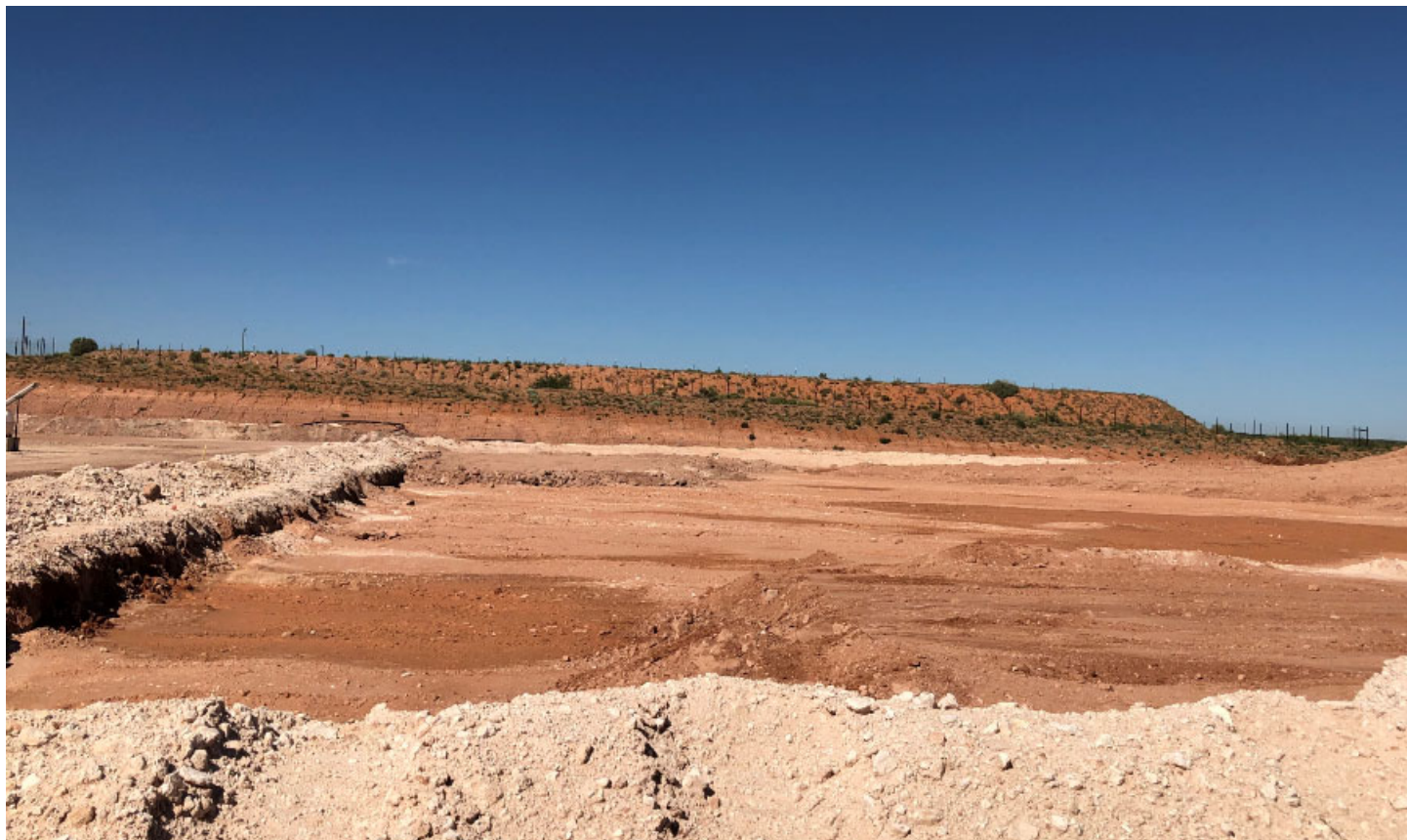
Figure 5 - Soil was placed over liner to hold in place.
