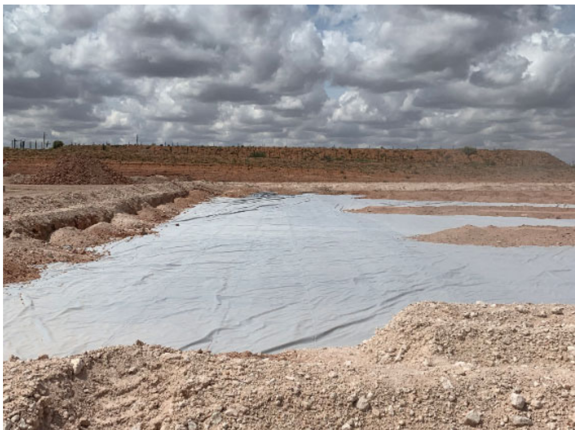
Figure 4 - Liner was placed (9/13/19)
