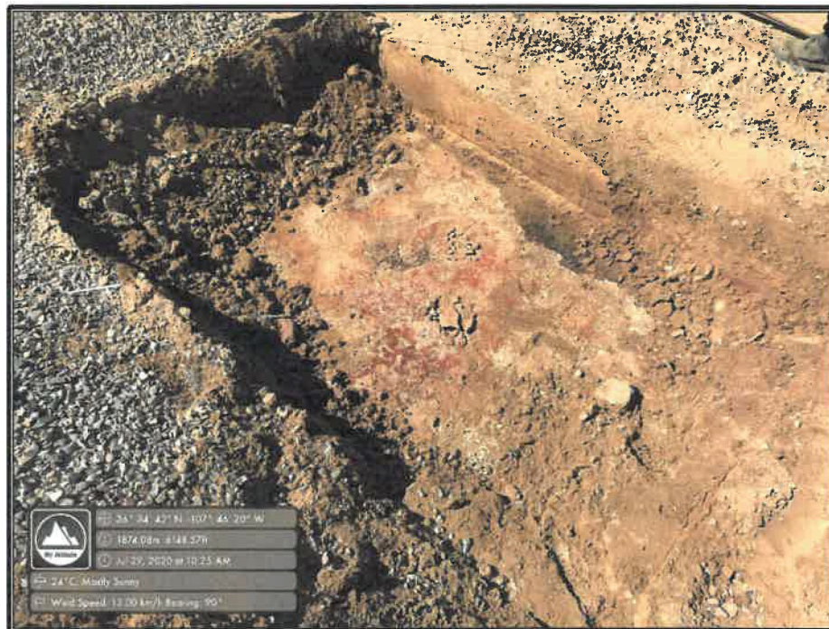
PHOTO 2: Former BGT Location after Removal (7/29/2020)
