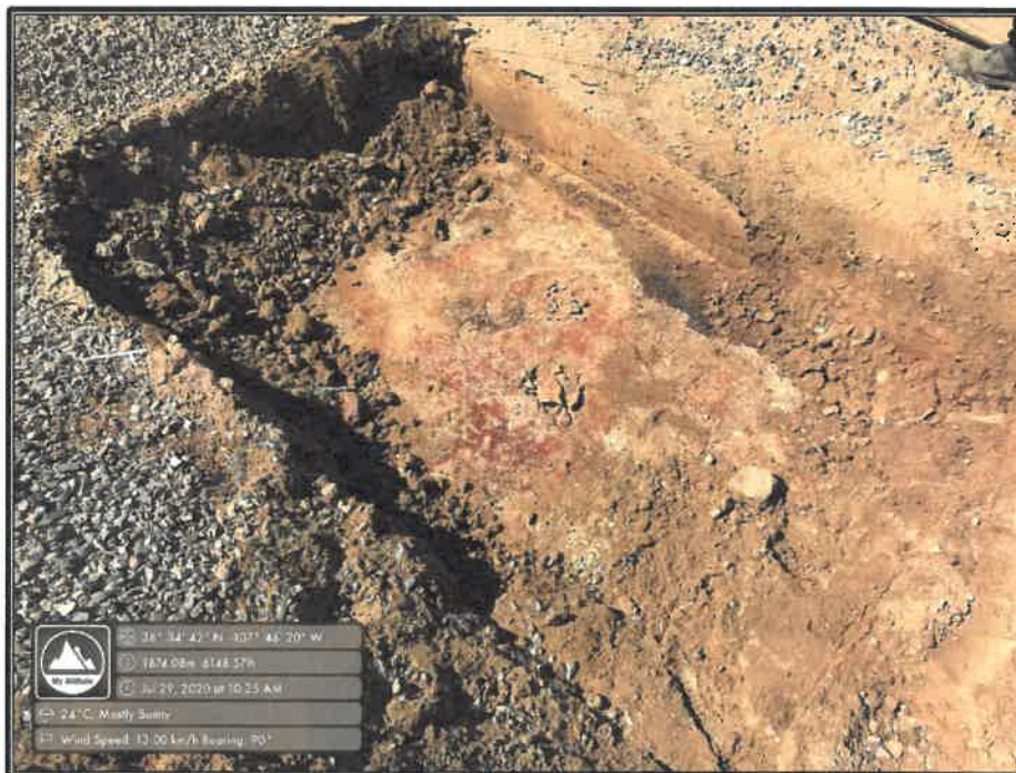
PHOTO 2: Former BGT Location after Removal (7/29/2020)
