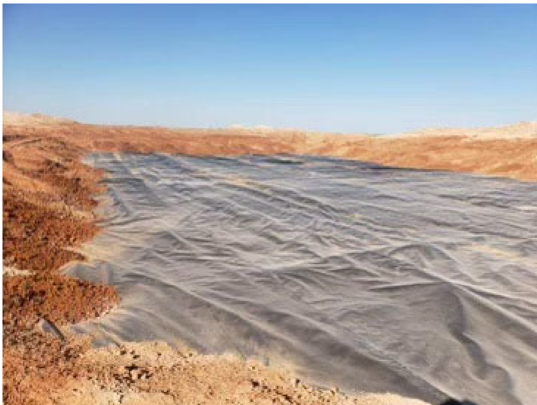
Photo 1: View of 40 mil HDPE liner within Temporary Pit
