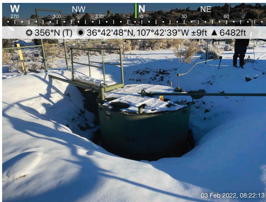
Photo 2: 45 bbls steel tank "A" prior to removal, 2/3/2022.
