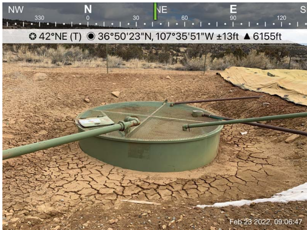
Photo 2: 40 bbls steel tank prior to removal, 2/23/2022.
