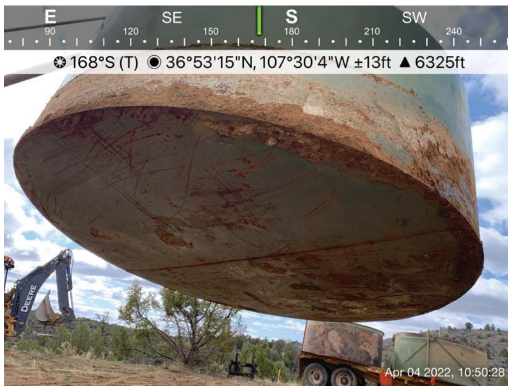
Photo 4: Bottom of BGT following removal, 4/4/2022.
