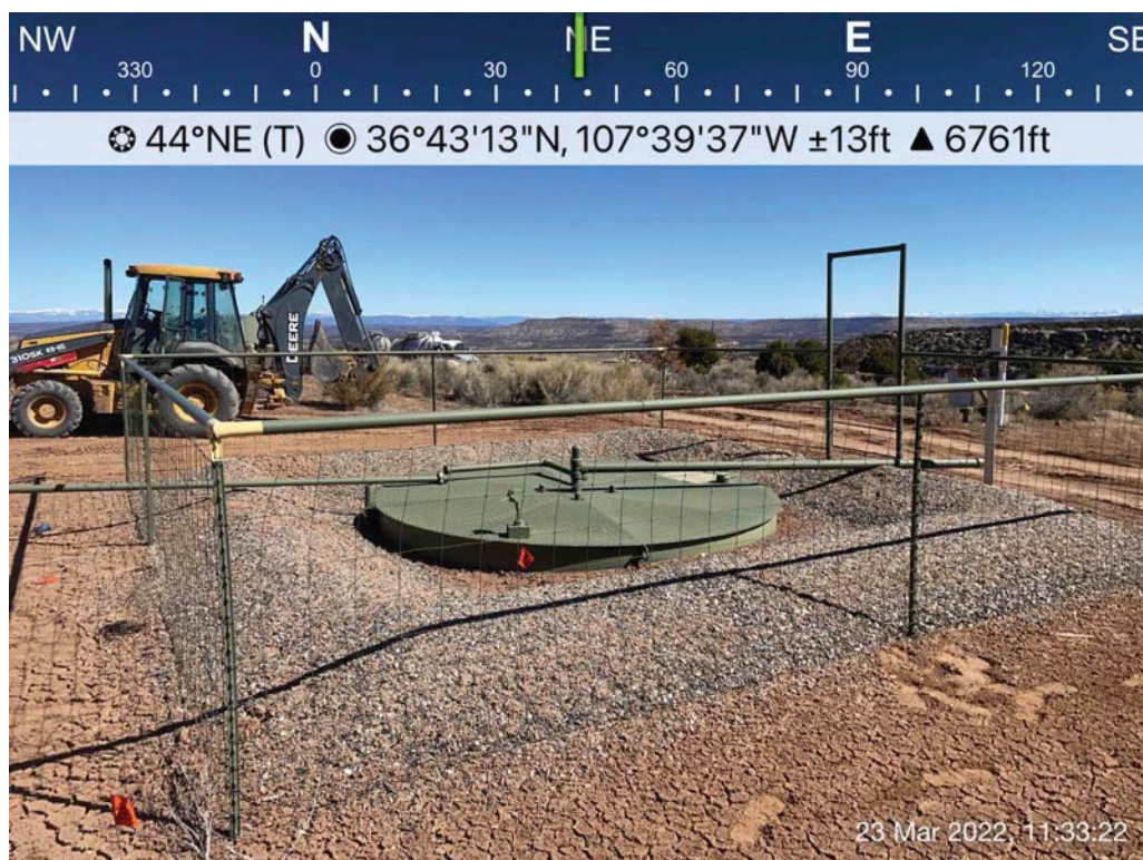
Photo 2: 95 bbls steel tank prior to removal, 3/23/2022.
