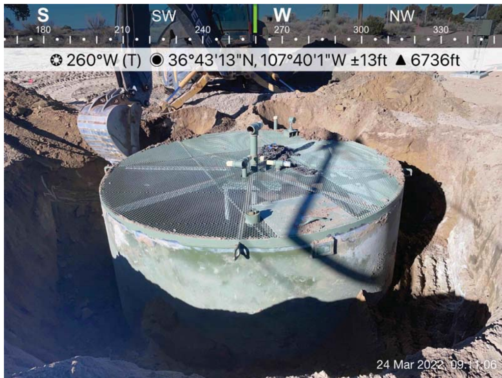
Photo 2: 95 bbls steel tank prior to removal, 3/24/2022.
