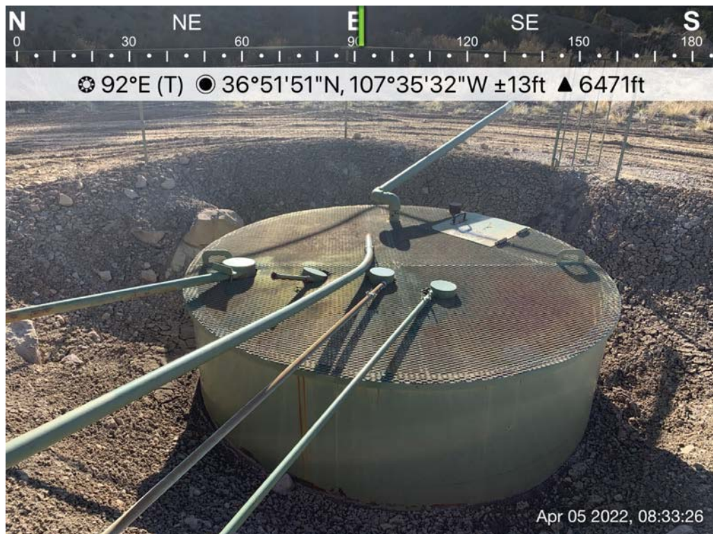
Photo 2: 40 bbls steel tank prior to removal, 4/5/2022.
