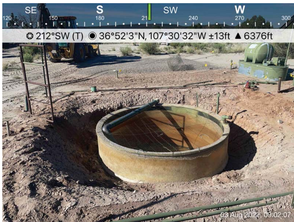
Photo 2: 35 bbls fiberglass tank prior to removal, 8/03/2022.
