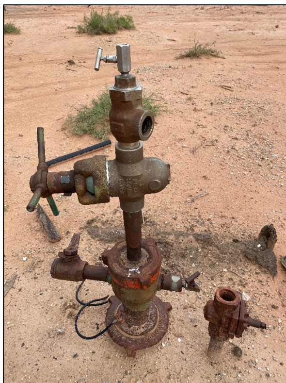
3) Twin Lakes SA #034L (30-005-60033) – Wellhead
