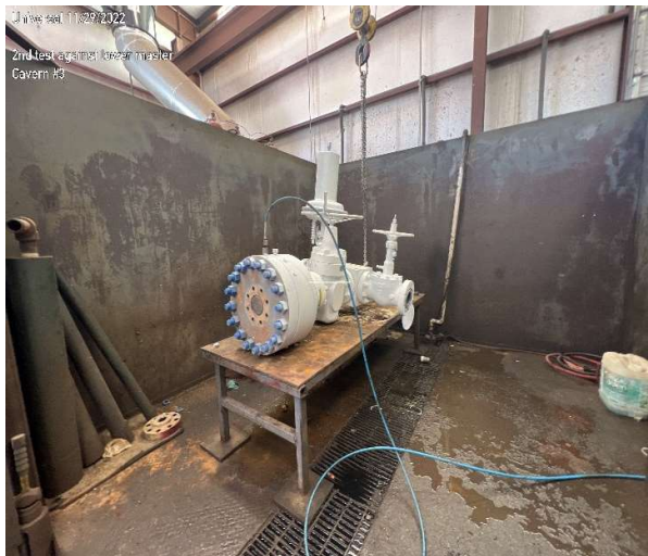
Well head with blind assembled with Teflon bolts for hydro testing
