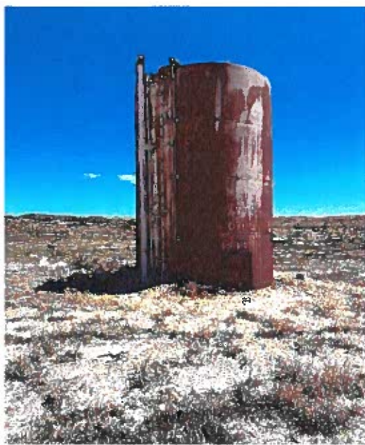
Photograph 7 Date: 5-9-2024 Description: 400 bbl AST and staining near valves View: East
