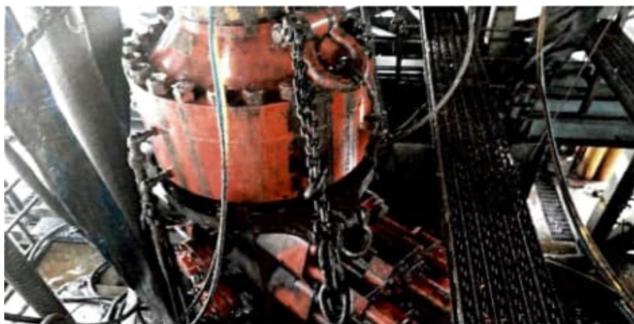
Figure 1: Winch System attached to BOP Stack
