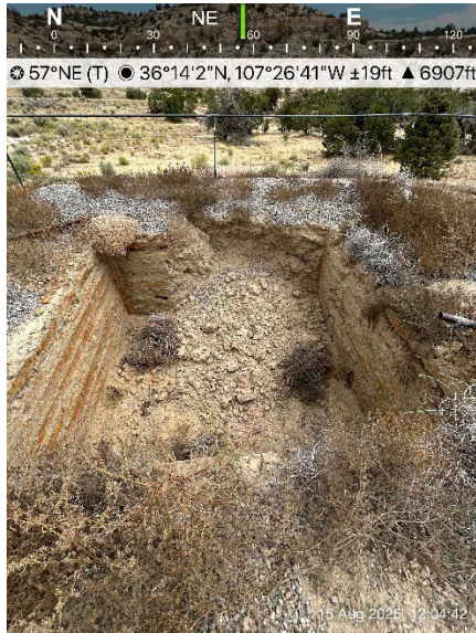
Photo 1: BGT after removal
