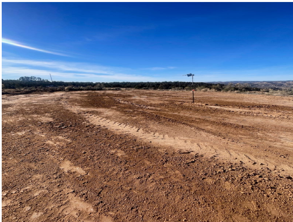
Photo 6: Former BGT location following backfilling and grading.
