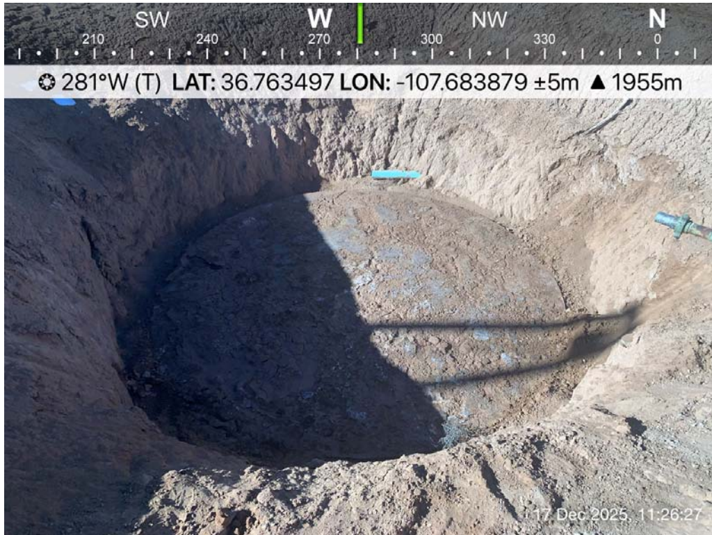
Photo 3: Location of BGT following removal.
