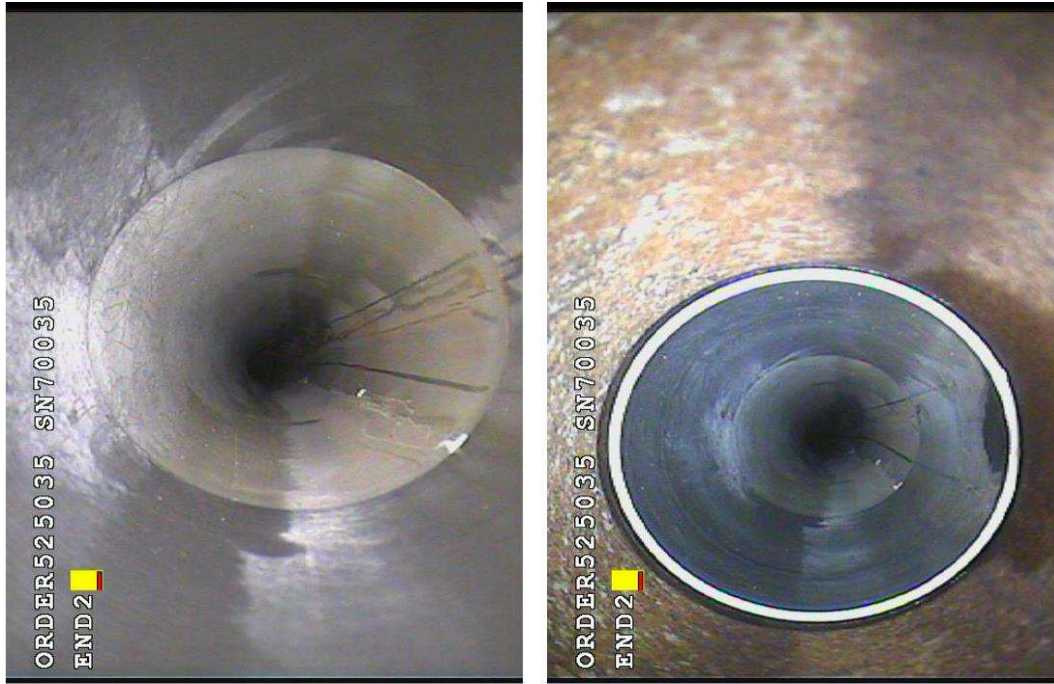
Photos: Liner/Coupling Interface END 2
