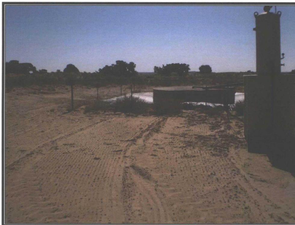
Photo 2: Excavated Area After Backfilling and Recontouring
