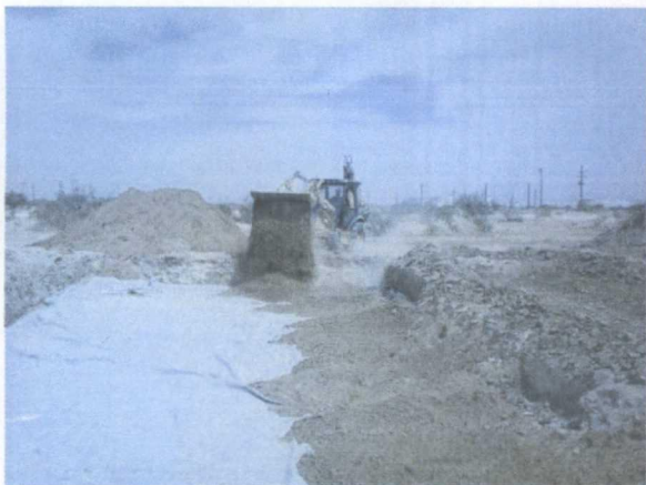
padding above the liner with 6" of blow sand, facing east
