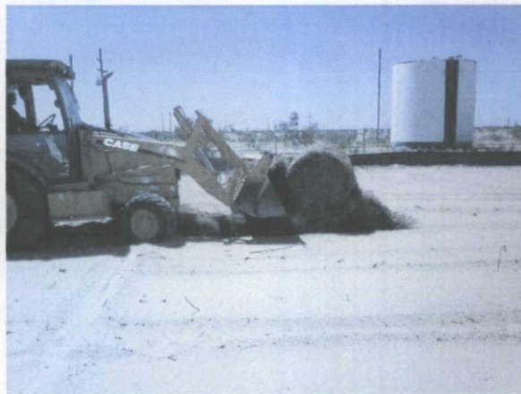
spreading peanut hay on the backfilled site, facing north
