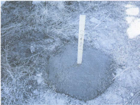
Completed plug and abandon
