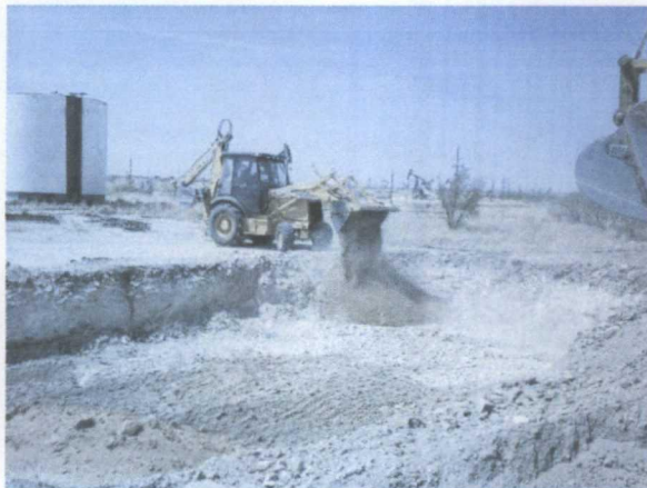
padding the base of the excavation with 6" of blow sand, facing west
