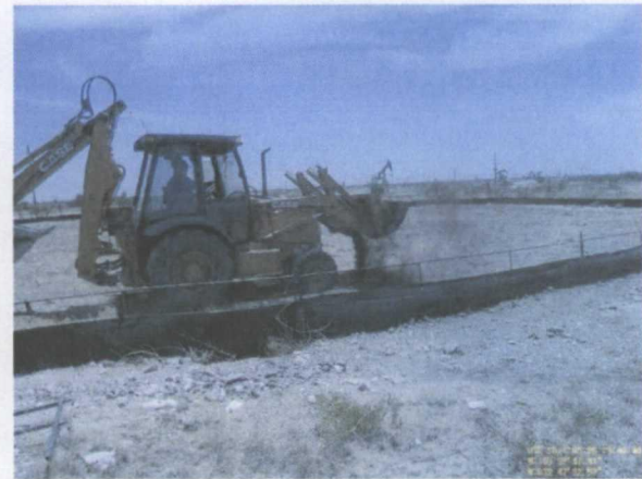
spreading bioNhance on the backfilled site, facing southwest
