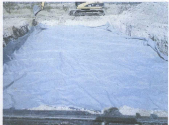
70x30 ft, 20-mil reinforced liner installed at 4 ft bgs, facing west
