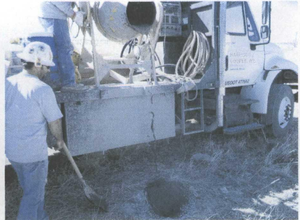
Plugging the bore with 1-3% bentonite/concrete slurry
