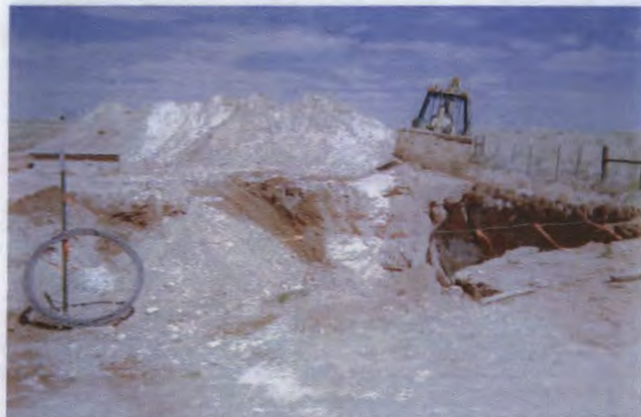
backfilling excavation site up to 6 ft BGS, facing north
