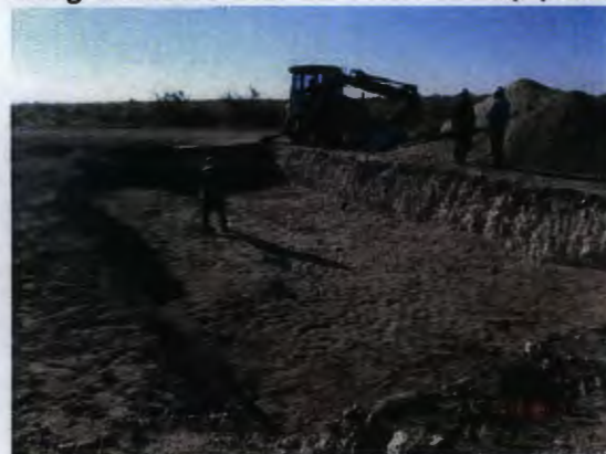
The bottom of the excavation padded with 6 inches of blow sand, facing southeast 6/10/2013
