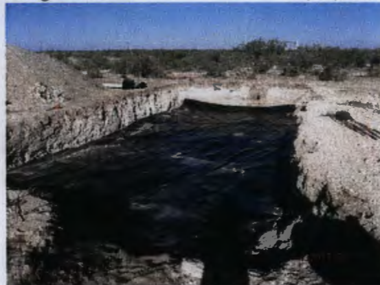
20-mil reinforced liner installed, facing southwest 6/11/2013
