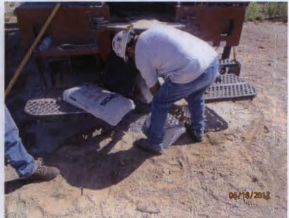
Plugging SB-1 in total with bentonite 6/18/13
