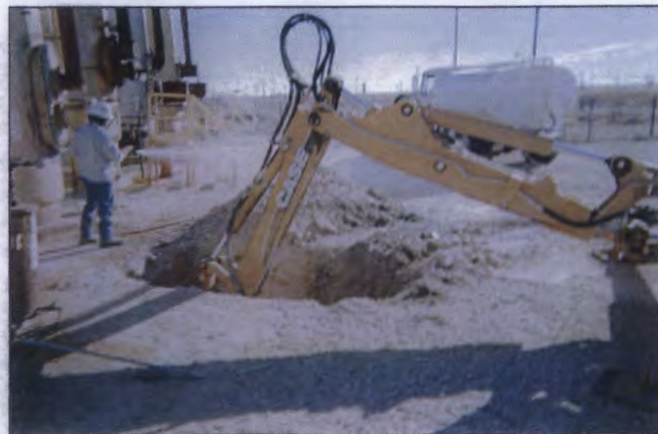
backfilling delineation trench
