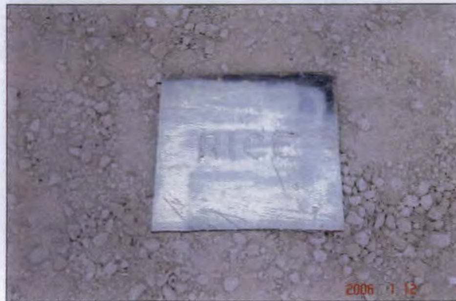
ID plate marking former junction box location
