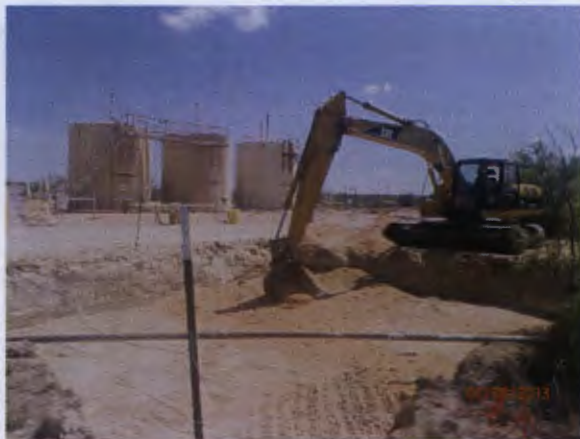
Installing 6" bottom sand pad, facing northeast 7/9/2013
