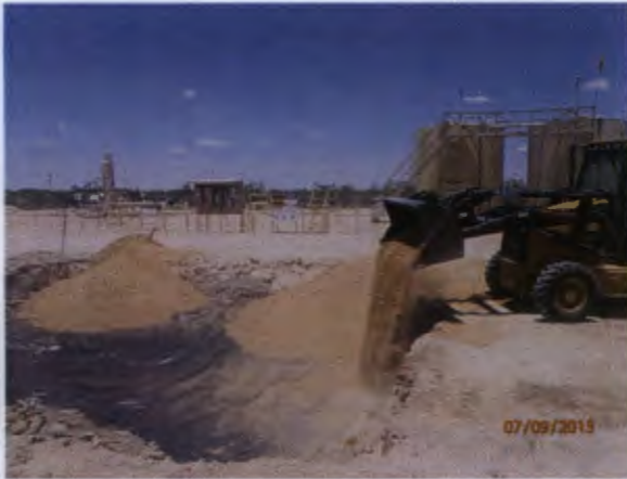
Padding liner with blowsand, Facing northwest
