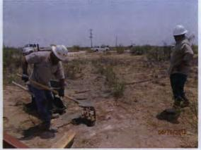
Plugging MW-1 with a 1-3% bentonite/concrete slurry and 3 ft concrete cap, facing north 6/19/13
