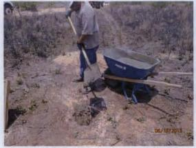
Plugging MW-2 with a 1-3% bentonite/concrete slurry and 3 ft concrete cap, facing north 6/19/13
