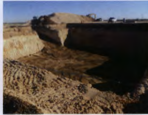
excavation complete to 27' bgs with a 6" blow sand pad installed, facing southeast
