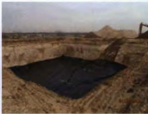
98'x98' 20 mil reinforced liner installed at 26.5', facing northeast
