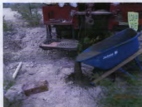
Plugging MW-2 with a 1-3% bentonite/concrete slurry with a 3 ft concrete cap, facing northeast 5/10/2013
