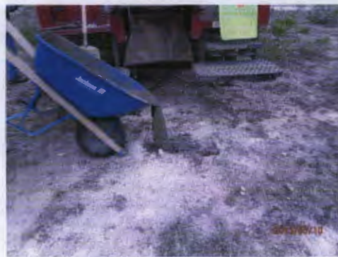
Plugging MW-4 with a 1-3% bentonite/concrete slurry with a 3 ft concrete cap, facing north 5/10/2013
