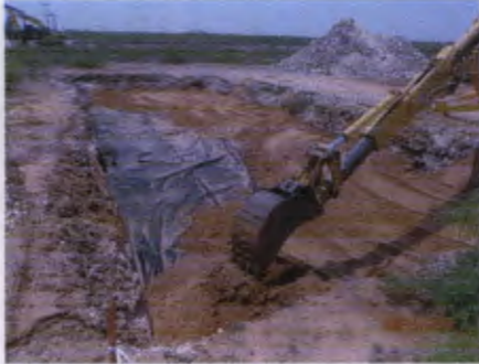
Padding liner with blowsand, Facing southwest 6/19/2013
