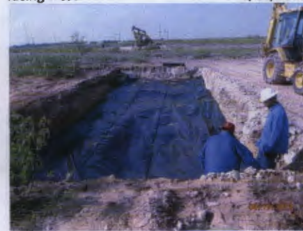
Installing liner, Facing south 6/19/2013
