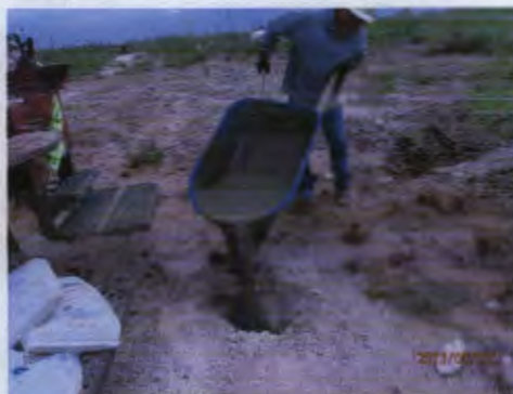
Plugging MW-1 with a 1-3% bentonite/concrete slurry with a 3 ft concrete cap, facing north 5/10/2013
