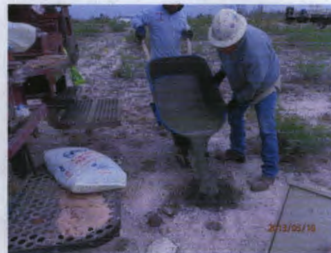
Plugging MW-5 with a 1-3% bentonite/concrete slurry with a 3 ft concrete cap, facing northeast 5/10/2013
