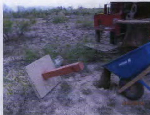
Plugging MW-3 with a 1-3% bentonite/concrete slurry with a 3 ft concrete cap, facing east 5/10/2013
