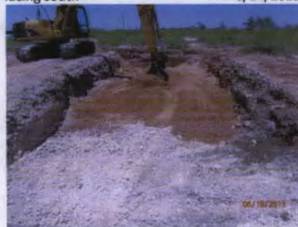
Installing 6" bottom sand pad, facing north 6/18/2013
