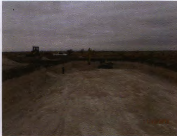
Excavating the southeast corner to a depth of 14 ft bgs, facing south 11/12/2013
