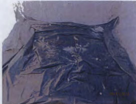
Installed 30'x30' liner @ 12' bgs
