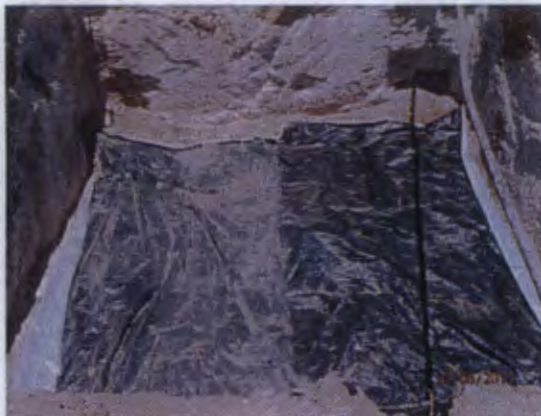
Installing 25'x25' liner at 12' bgs
