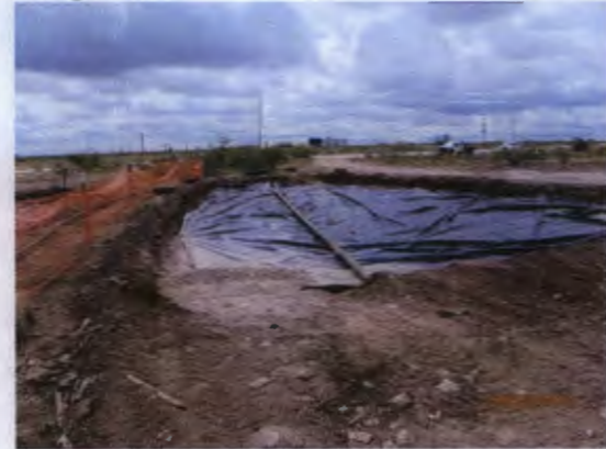
20-mil, reinforced liner installed, facing southwest
