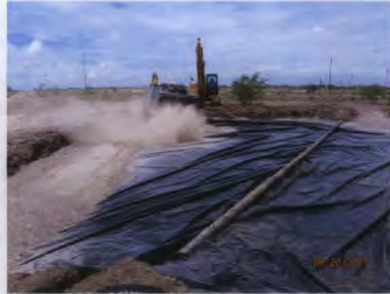
Padding above the liner with pond bottom, facing east 9/20/2013
