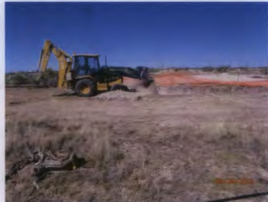
Padding the second 20-mil, reinforced liner with pond bottom and backfilling, facing east 9/24/2013
