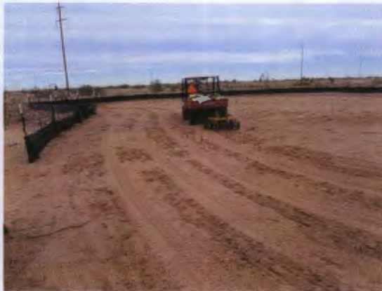
Discing the backfilled excavation, facing west 10/30/2013
