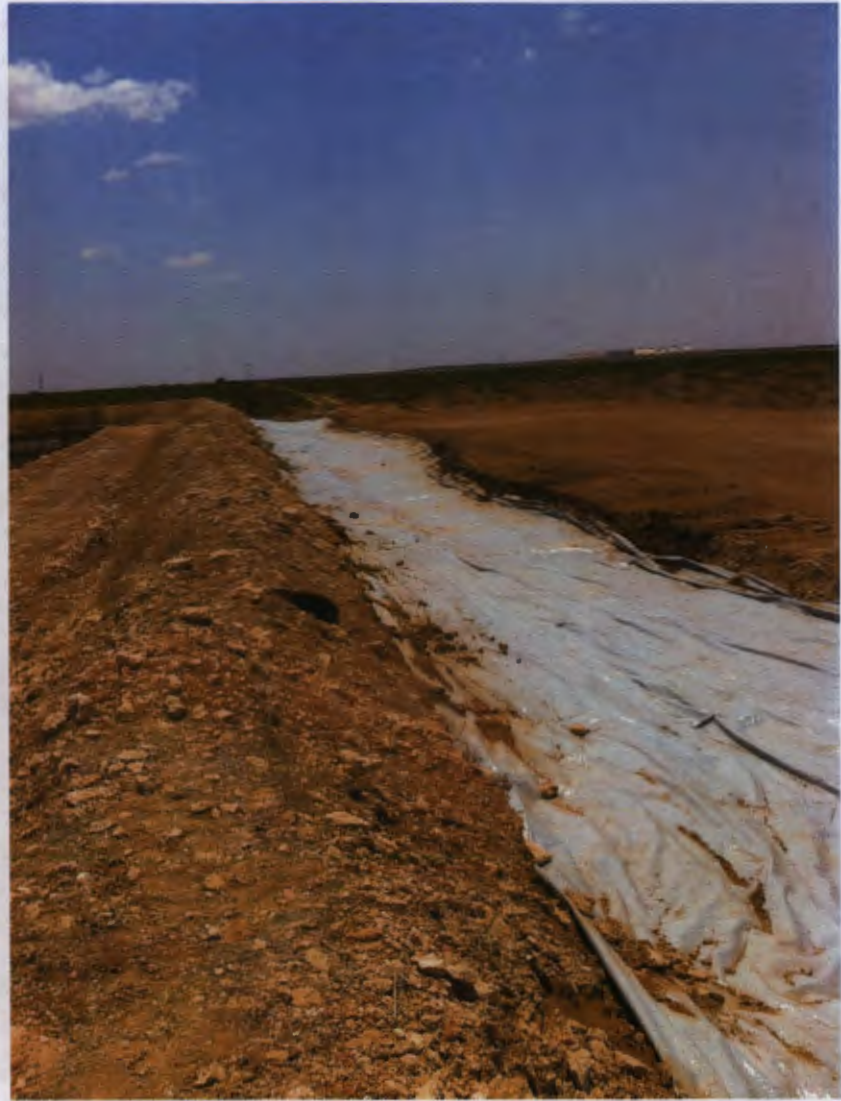
Completed liner installation, with liner keyed into the facility berm
