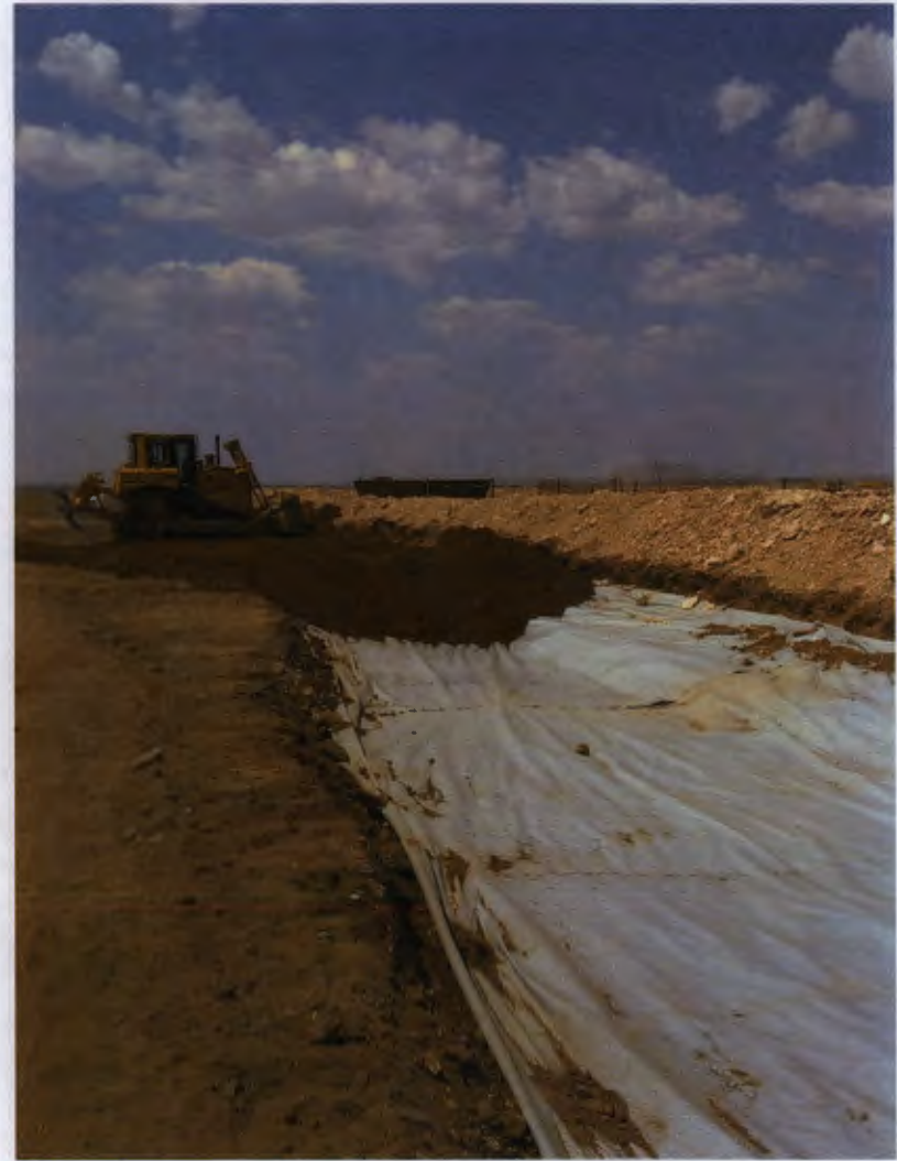
Pushing clean fill over the liner
