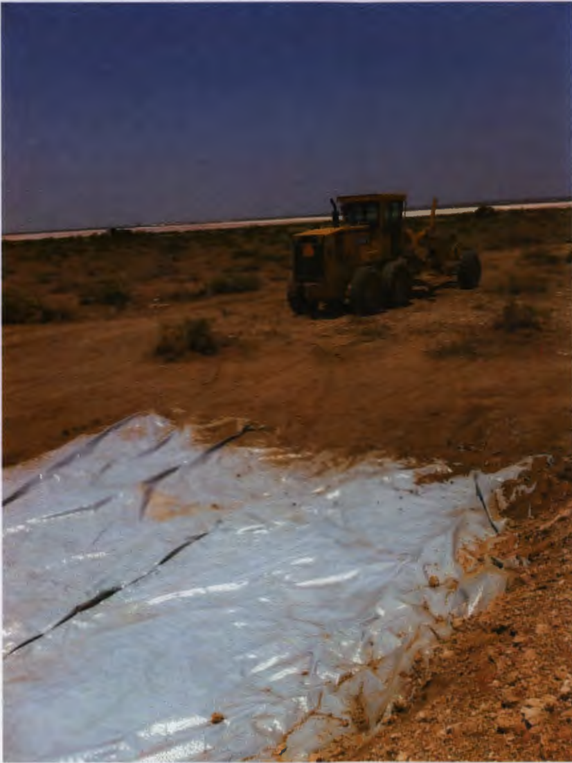
North end of the installed liner
