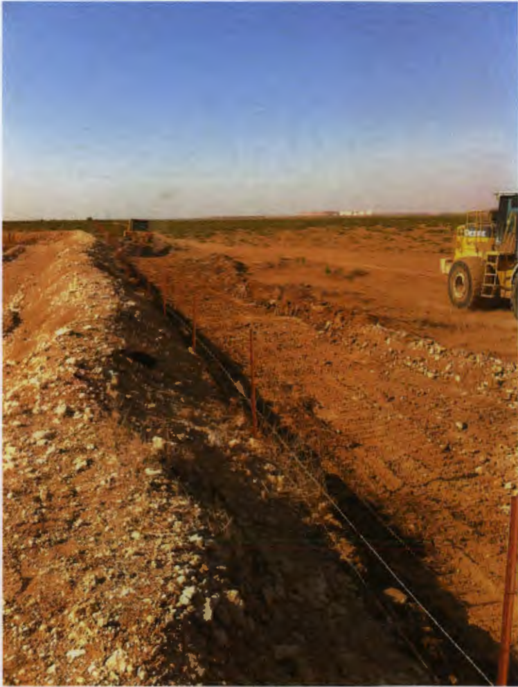
Initial excavation cut
