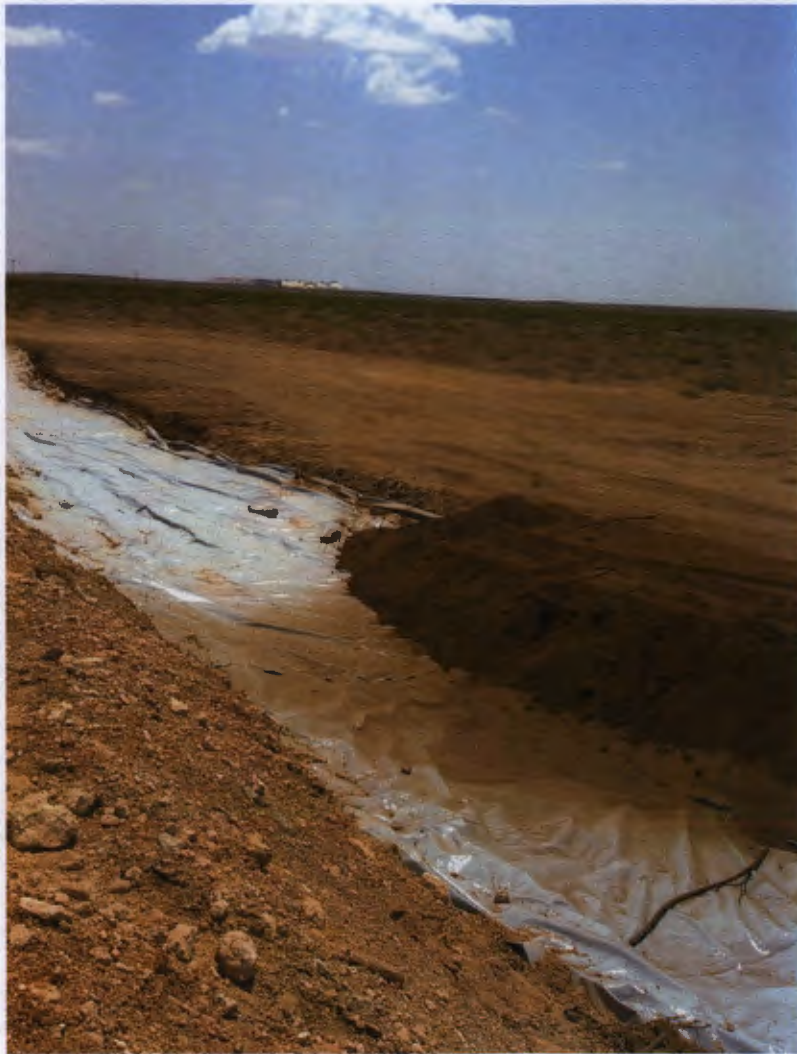
Initial placement of clean fill material
