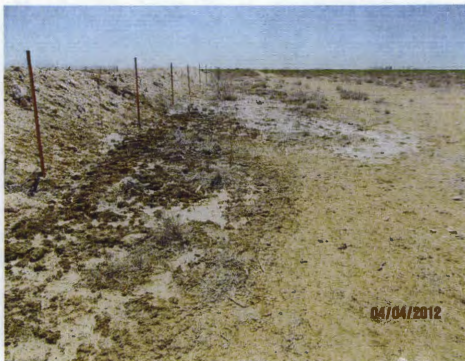
3. Spill Area Viewing South, April 4, 2012
