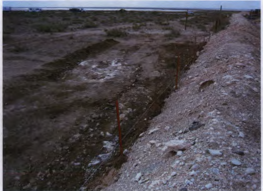
Excavation work at the end of day 1
