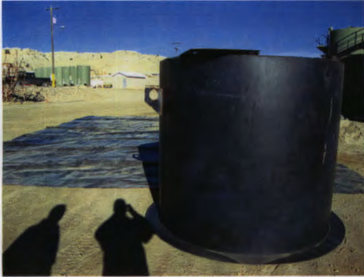
New Double Walled Tank
