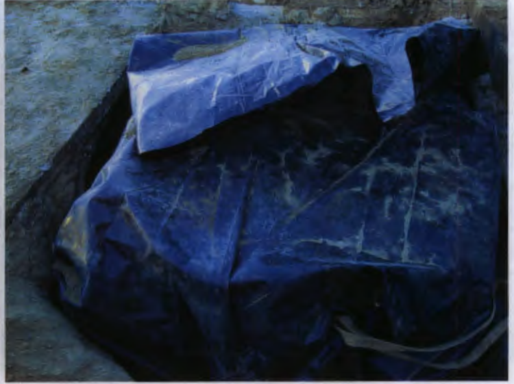
New Double Walled Tank wrapped in a liner
