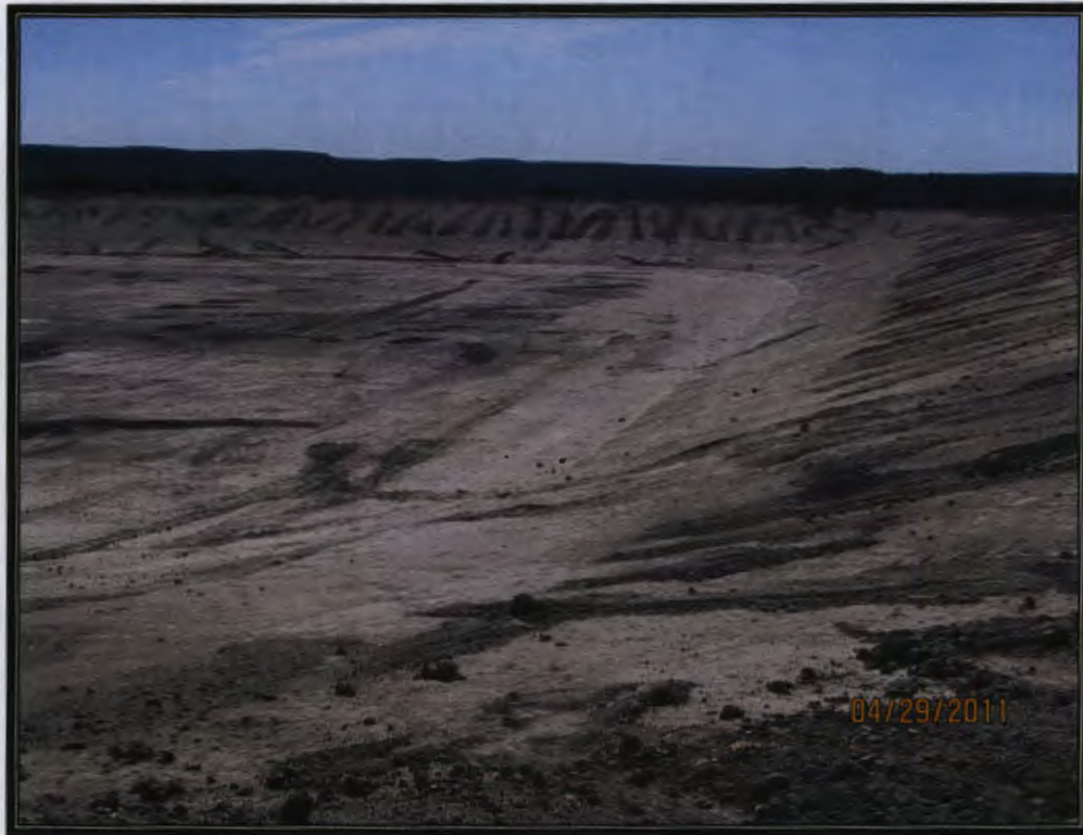
Photo 5: Pond after Liner Removal
