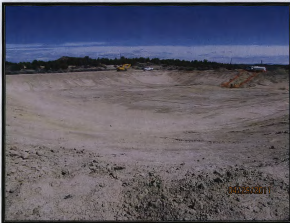
Photo 5: Pond after Liner and Leak Detection Removed
