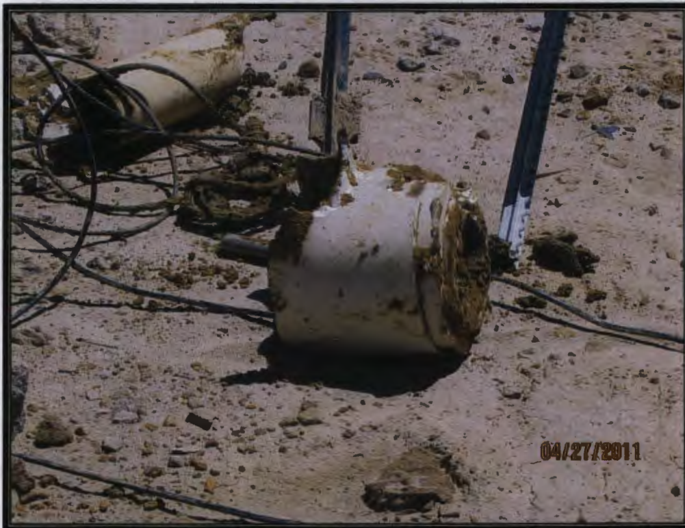
Photo 4: Bottom of Leak Detection System, 8" PVC, No Concrete Sump Found
