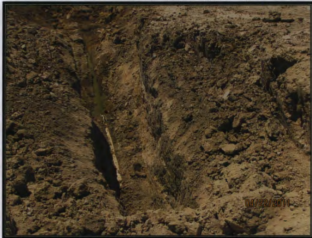
Photo 2: Removing the Leak Detection System
