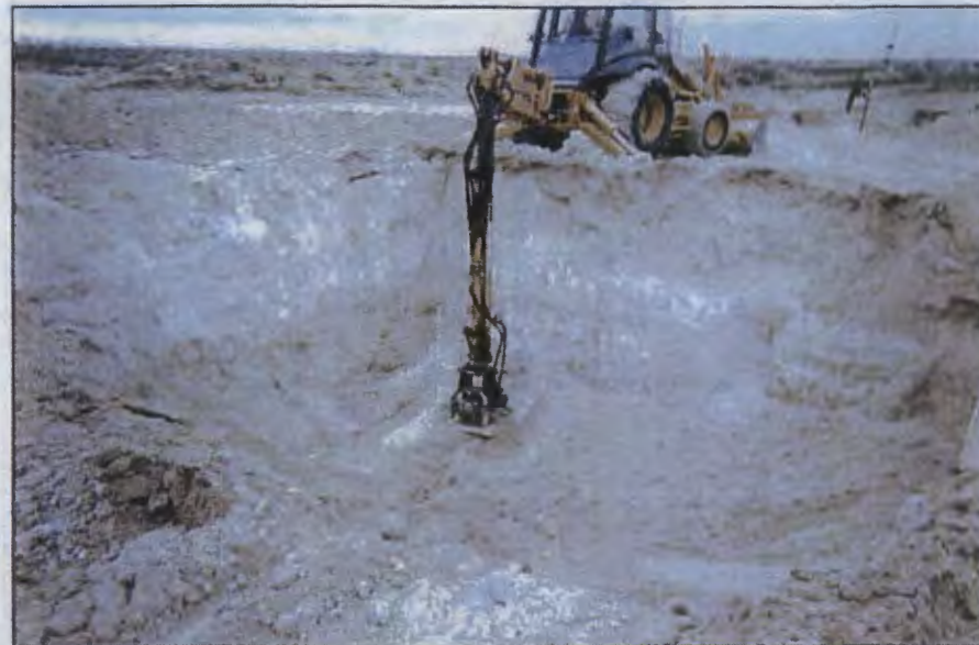
compacting backfill in 25 x 20 x 12 ft excavation 1/29/2007
