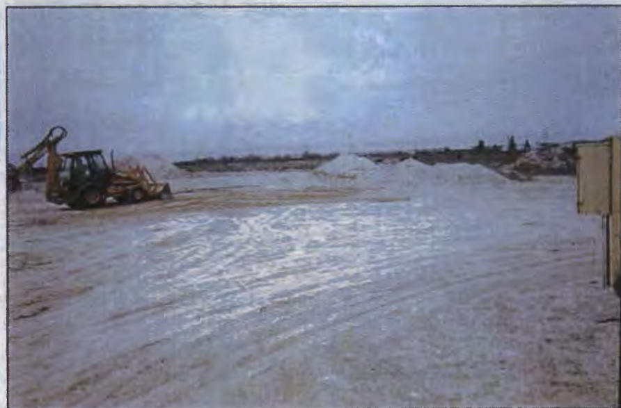
spreading clean, imported soil on top of backfilled site 1/30/2007
