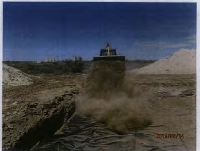
Backfilling 2 nd Liner, facing east 8.14.13
