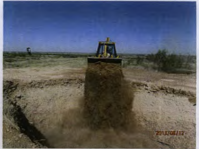
Backfilling Liner, facing west 8.12.13
