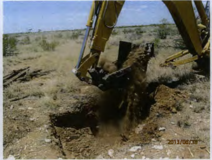
Digging vertical, facing north 6.18.13
