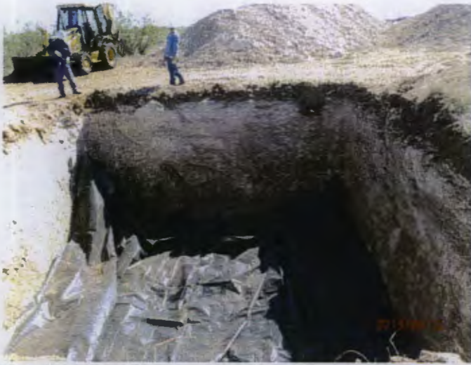
Installing 20 mil liner at 12ft bgs, facing east 8.12.13
