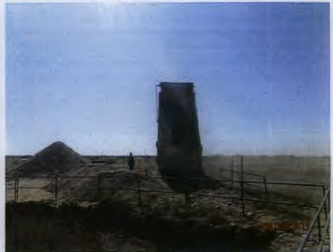
Importing soil, facing east 8.9.13
