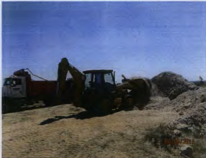
Exporting soil, facing south 8.9.13
