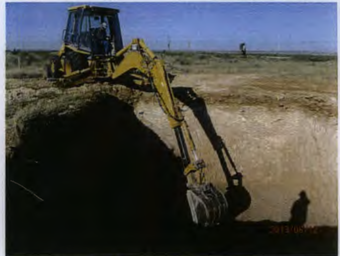
Padding bottom of excavation, facing west 8.12.13
