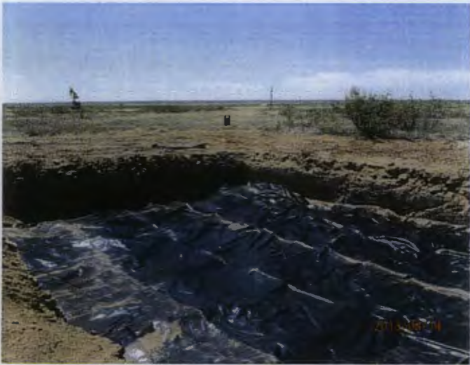
Liner installed 5'ft bgs below ground surface, facing northwest 8.14.13
