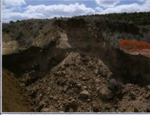
Description: View of the southwest portion of the excavation with restricted access because of steep slope and sloughing.
