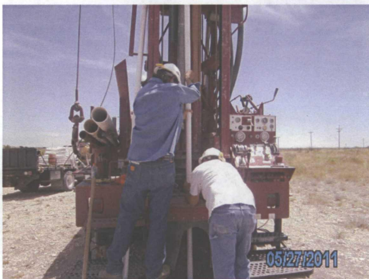
Inserting the 2 in casing, facing S
