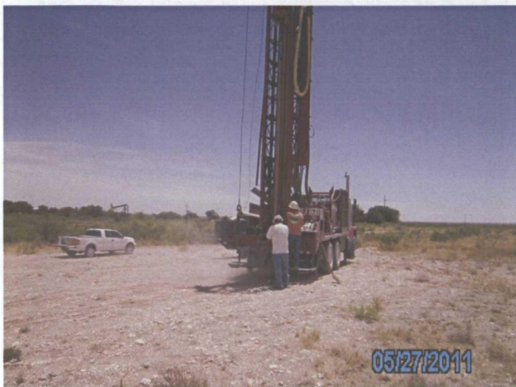
Drilling the soil bores, facing SE
