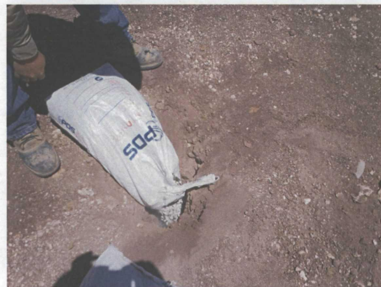
Plugging the SB in total with bentonite
