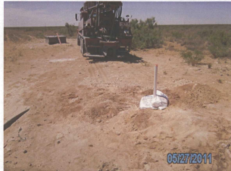
Packing the top of the bore with bentonite 5/27/2011
