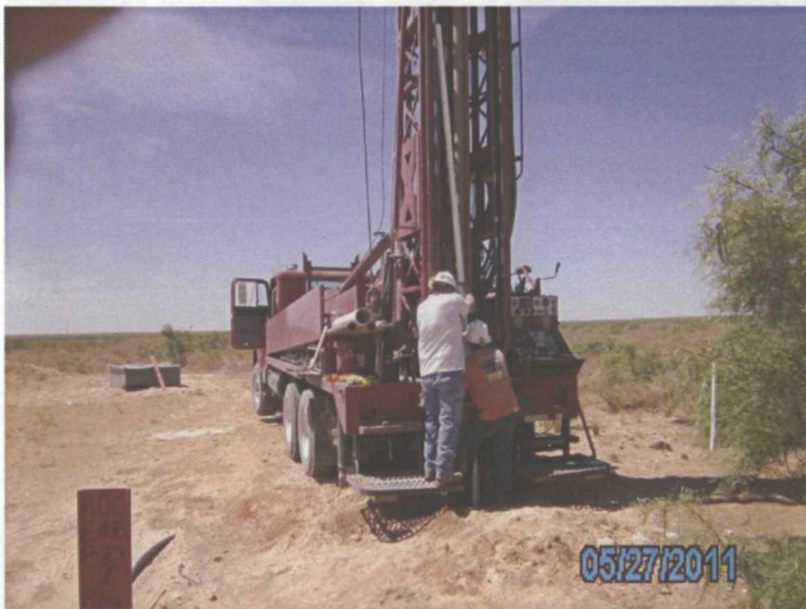
Inserting 2 in casing into well, facing S
