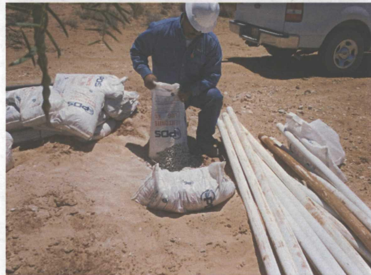
Plugging the SB in total with bentonite
