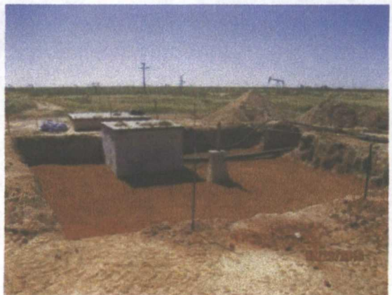
excavation padded with sand, facing southwest
