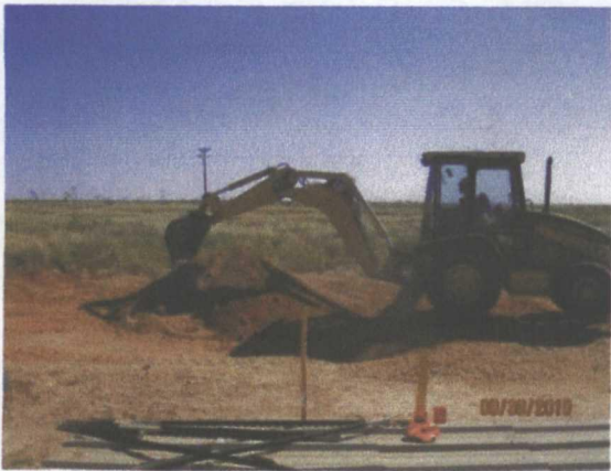
blending backfill, facing east
