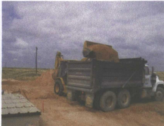
hauling off soil, facing
