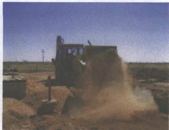
backfilling with hay-soil mix, facing southwest
