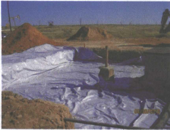
plastic liner installed, facing east
