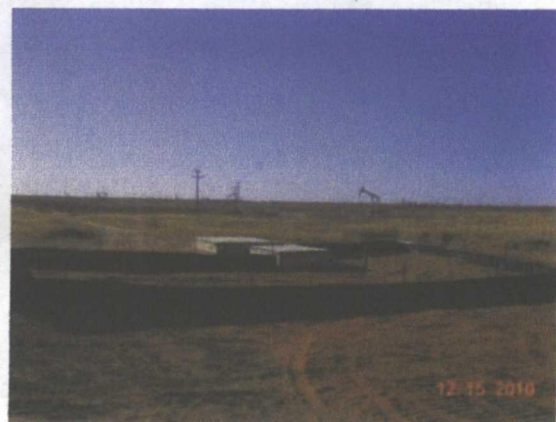
site completed, facing south
