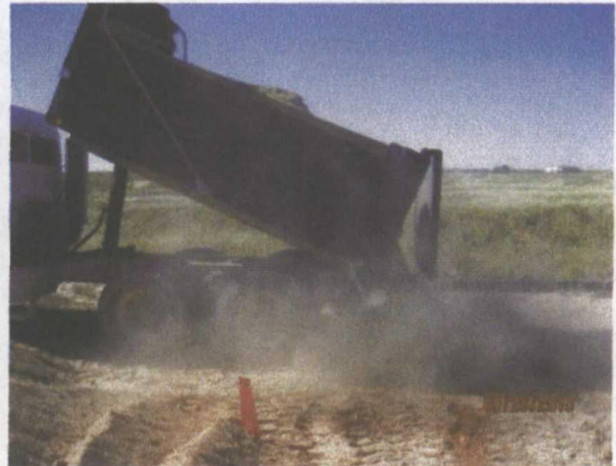
hauling in hay-soil mix, facing west
