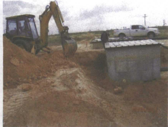
excavating, facing south
