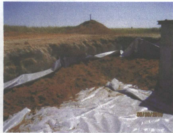
padding on top of plastic liner, facing southwest
