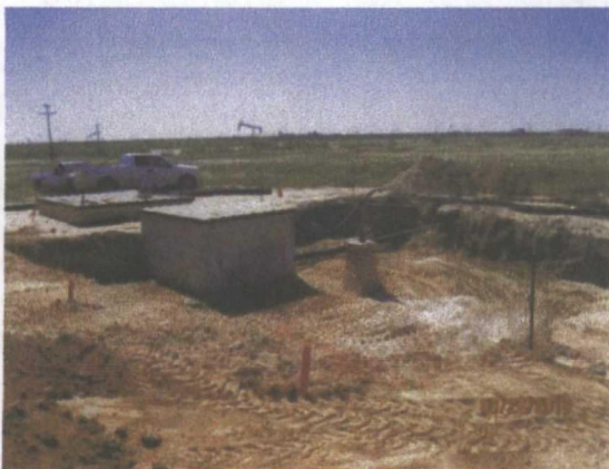
excavation completed, facing southwest
