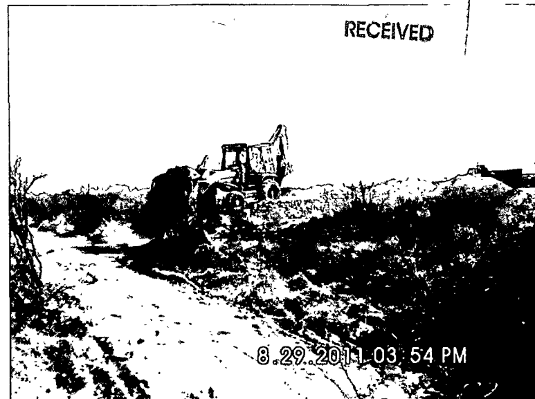
Backfilling the site, facing southeast
