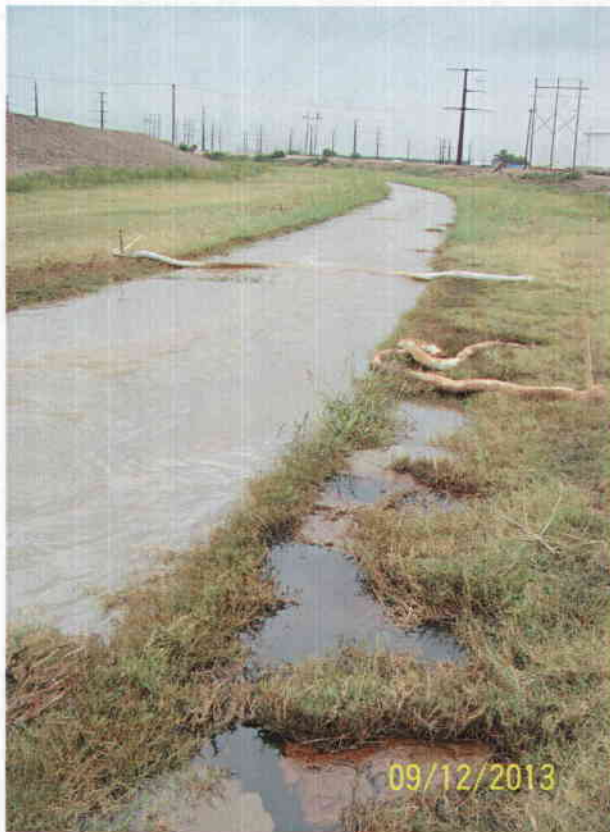
Looking east from Freeman St. crossing – Boom across Eagle Draw, booms used to soak up eddied oil
