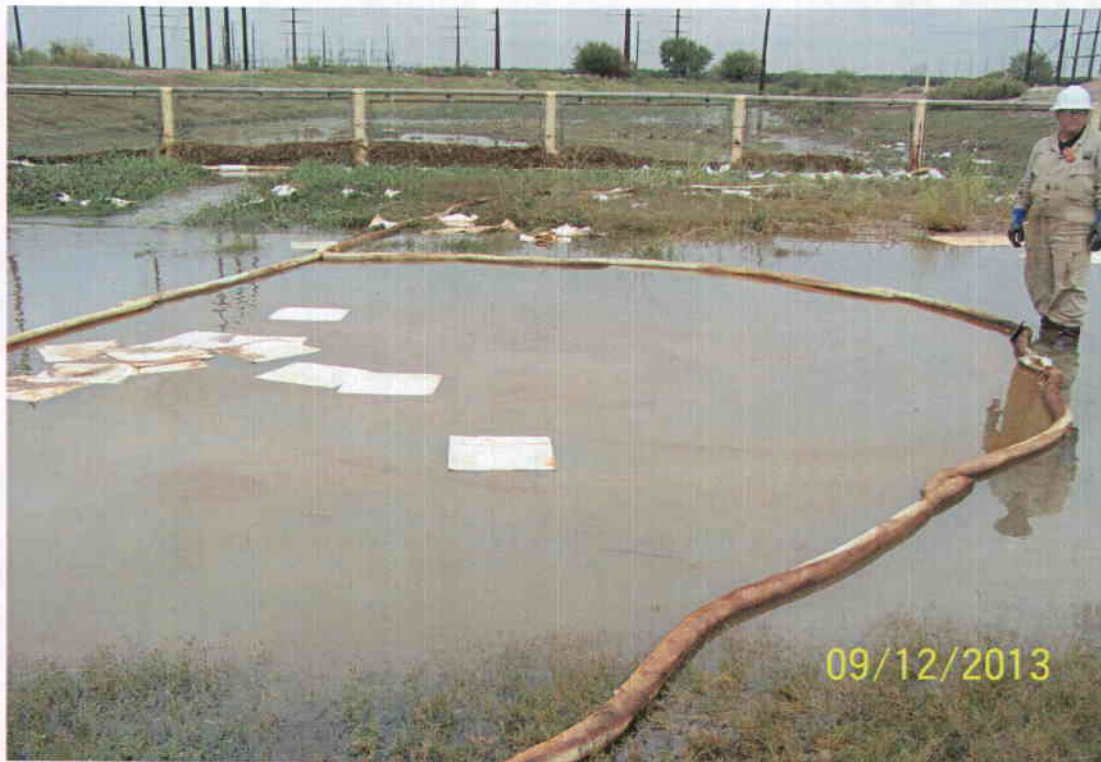
5 th St. crossing – oil sheen in trap, oil sorbent pads skimming
