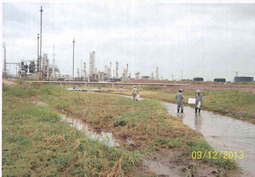
Eagle Draw further downstream – Mopping up with oil sorbent pads
