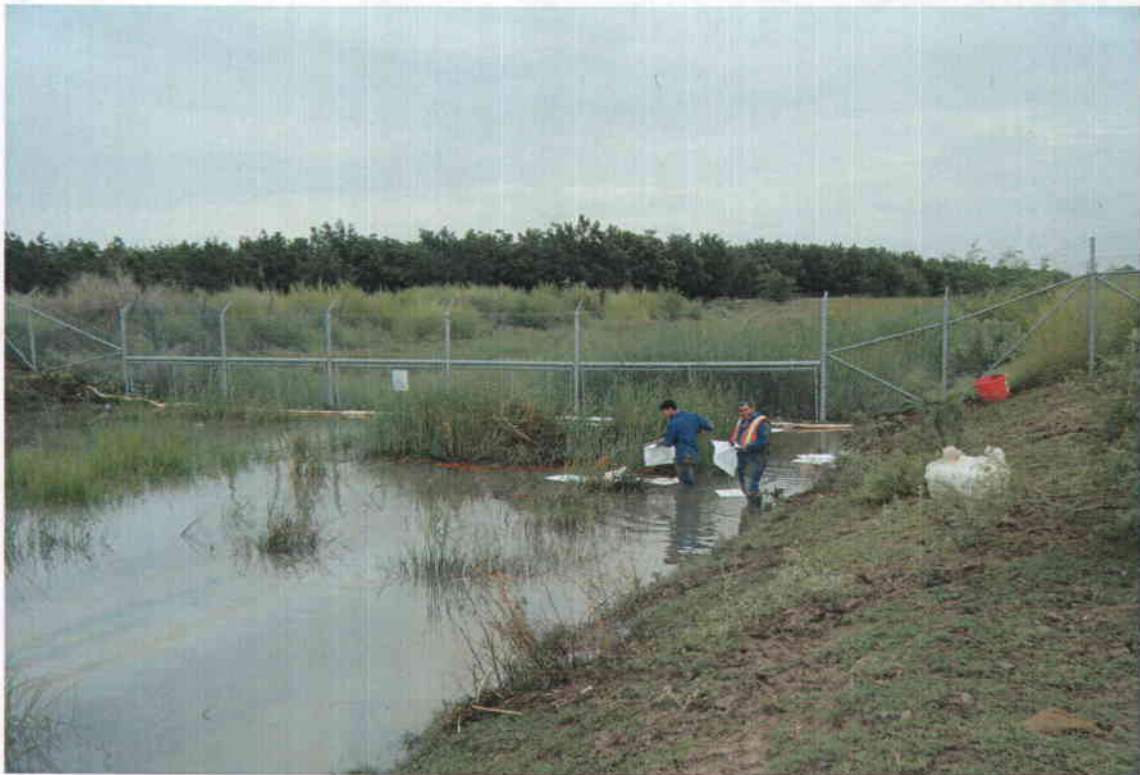
Farm Field Fence – Navajo property both sides – Using oil sorbent pads to capture sheen
