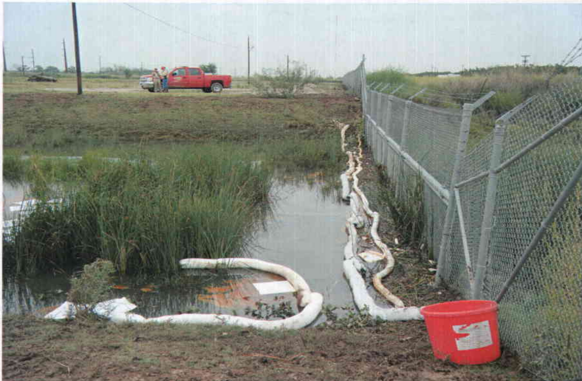
Farm Field Fence – Navajo property both sides – Boom and trap arrangement
