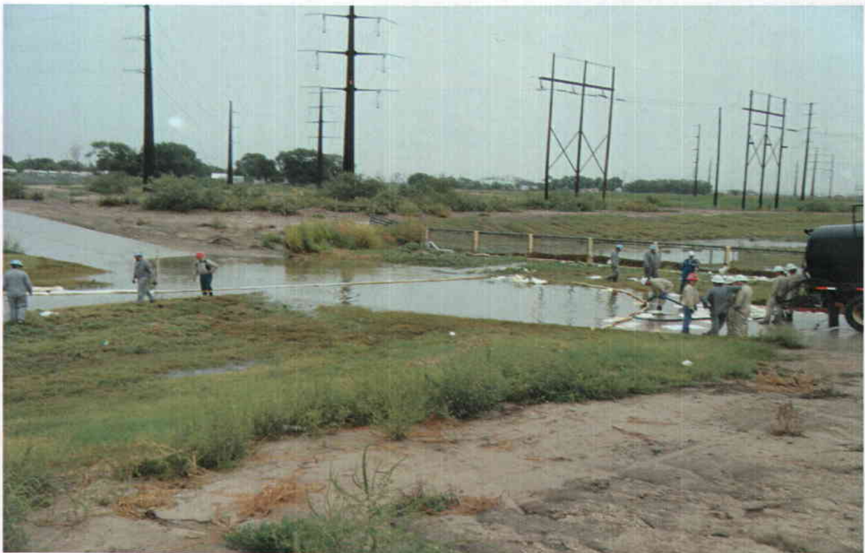
5 th St. Crossing – Boomed oil trap, oil-only skimmer pads, vacuum truck – west of cow pasture fence
