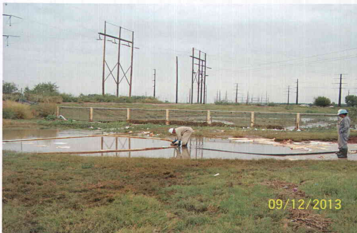
5 th St. crossing – suctioning oil trap with vacuum truck hose
