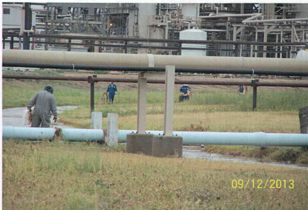
Eagle Draw east of spill – Mopping up with oil sorbent pads and socks
