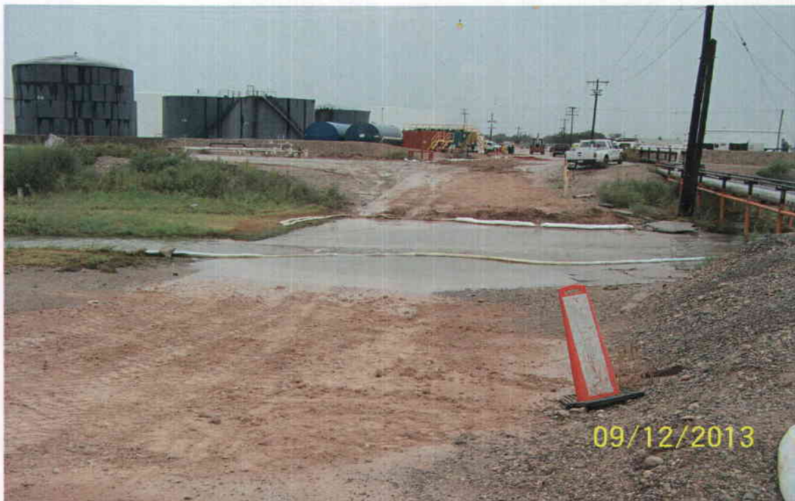
Freeman St. crossing – Site of release to Eagle Draw – Sand placed on concrete pavement to prevent oil movement to Eagle Draw. Booms placed to capture oil in eddies.
