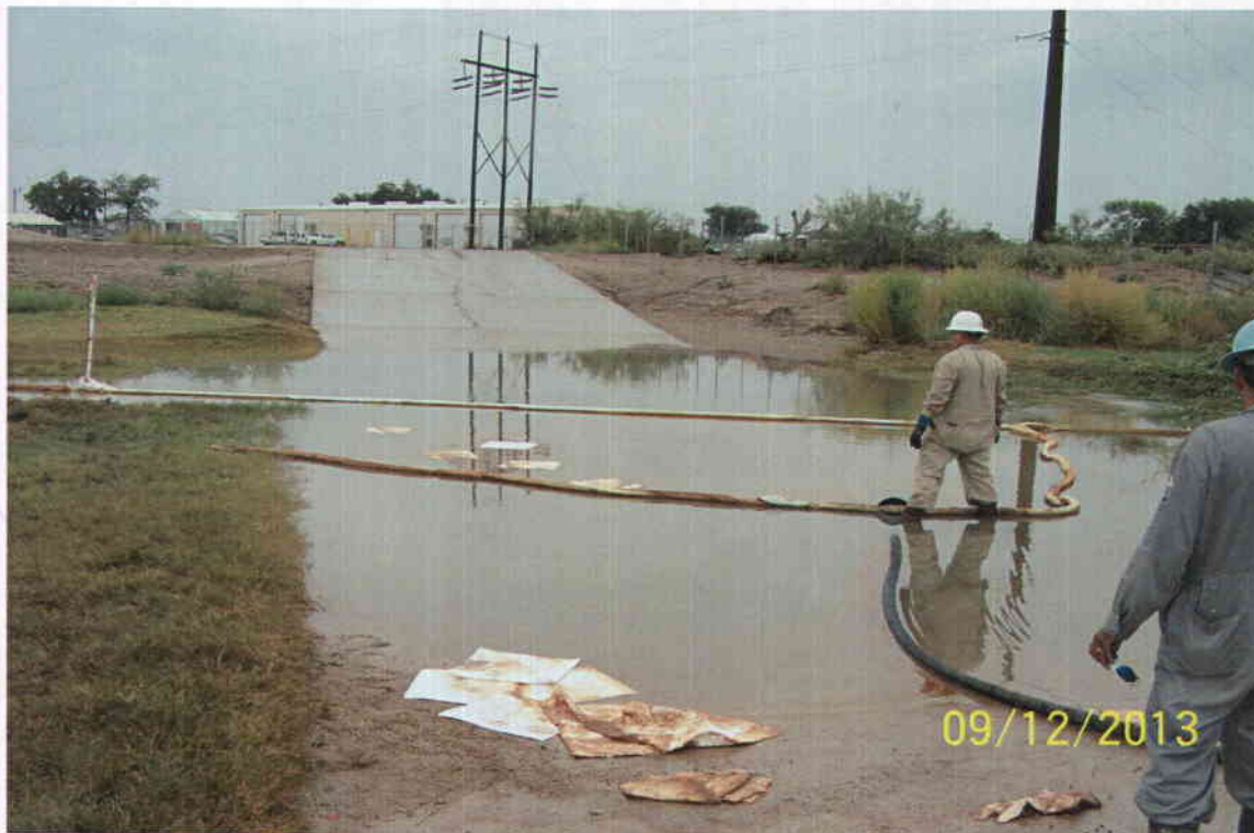
5 th St. crossing – oil trap and vacuum truck suctioning, oil sorbent pads skimming
