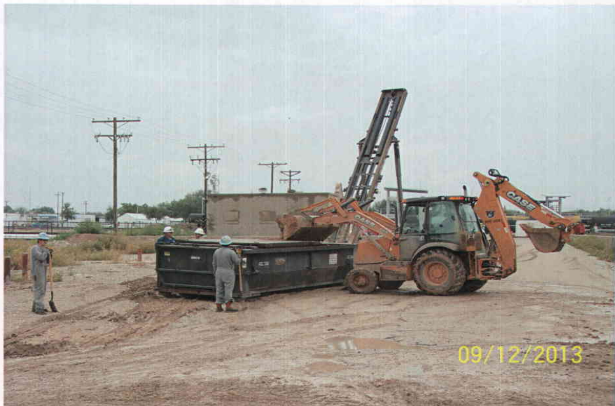
Freeman St. – scraping sand from pavement into a rolloff bin
