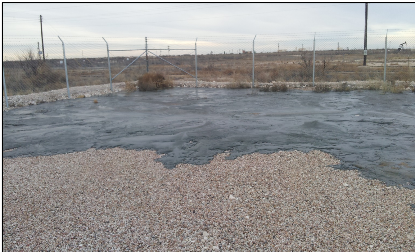
Photo 3: Gas oil retained within diked containment southeast of release (December 27, 2012).
