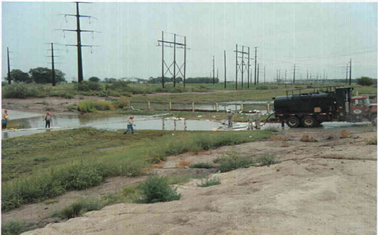
5 th St. Crossing – Boomed oil trap, oil-only skimmer pads, vacuum truck – west of cow pasture fence
