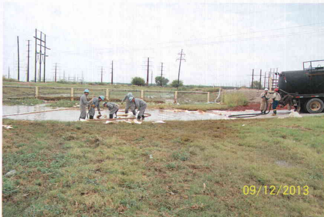
5 th St. crossing – finishing skimming by hand with oil sorbent pads
