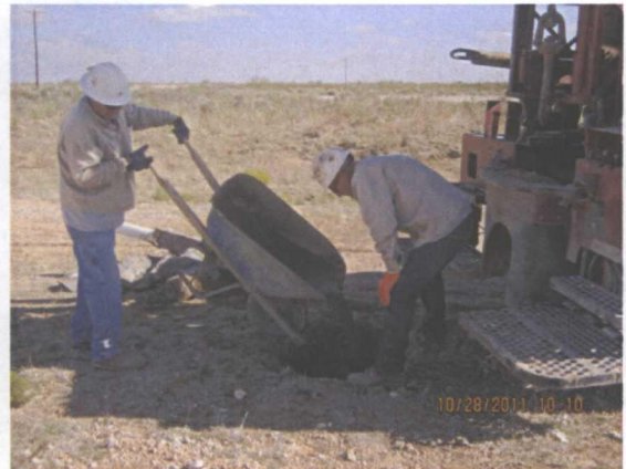
Plugging the bore with 1-3% bentonite/concrete slurry, facing north 10/28/11
