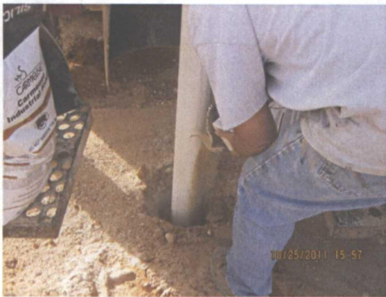
Inserting the sand pack 10/25/11
