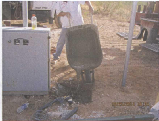
Plugging MW-2 with a 1 – 3% bentonite/concrete slurry
