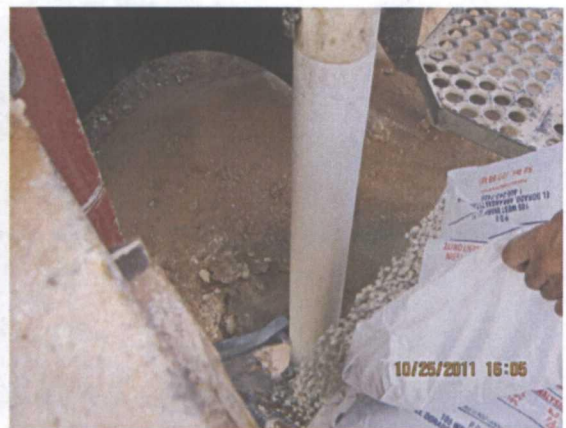
Inserting the bentonite seal 10/25/11
