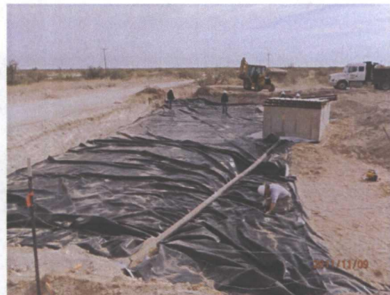
installing the north half of the 20-mil reinforced liner, facing east
