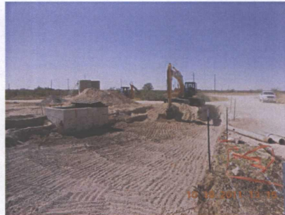
excavating the site, facing east
