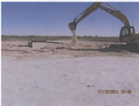
backfilling the excavation, facing east
