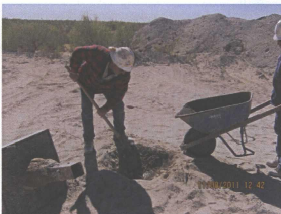
Plugging MW-3 with a 1 – 3% bentonite/concrete slurry, facing south 11/8/11
