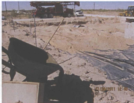
Plugging MW-1 with a 1 – 3% bentonite/concrete slurry, facing northwest 11/8/11
