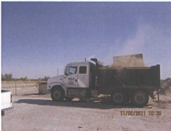
exporting excavated soil, facing east
