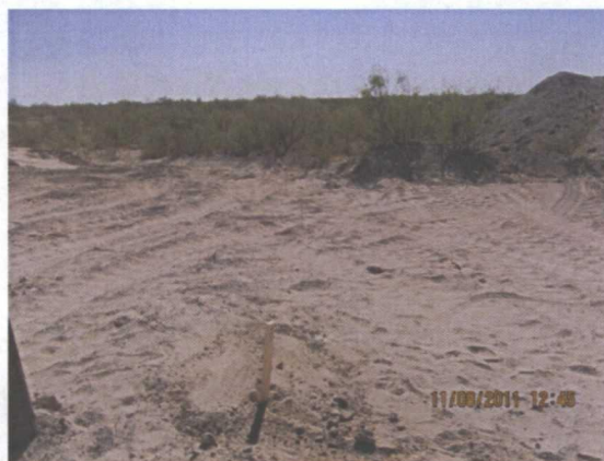
MW-3 plugged, facing south 11/8/11
