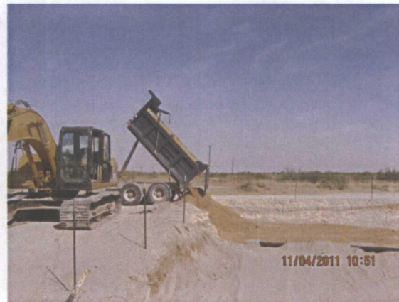
importing blow sand to pad the excavation, facing north
