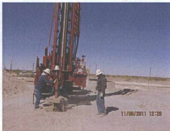
Pulling MW-3, facing northwest 11/8/11
