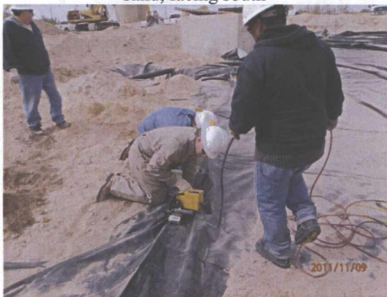
fusing the north and the south liners, facing west
