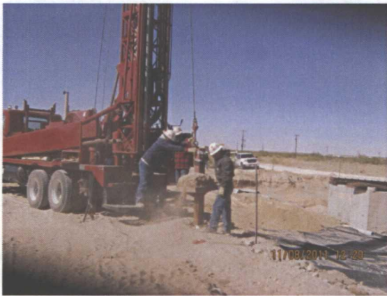
Pulling MW-1, facing northwest 11/8/11
