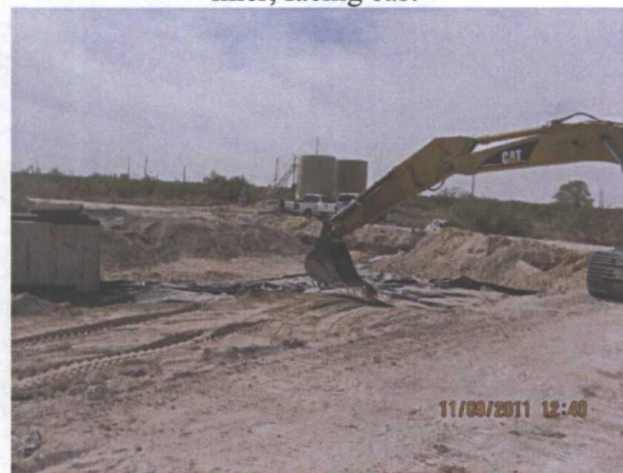
padding the north liner with 6 inches of blow sand, facing southwest
