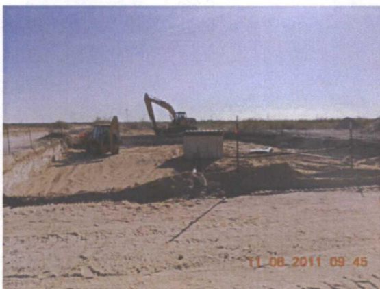
73x98 ft excavation complete with a 6 inch blow sand pad, facing east
