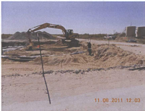
padding the south liner with 6 inches of blow sand, facing south
