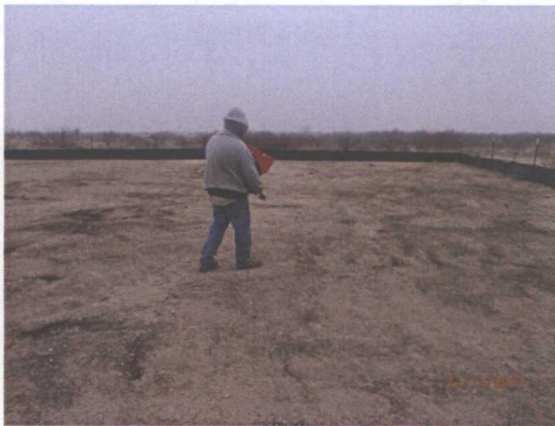
seeding the backfilled site with blue grama, facing east
